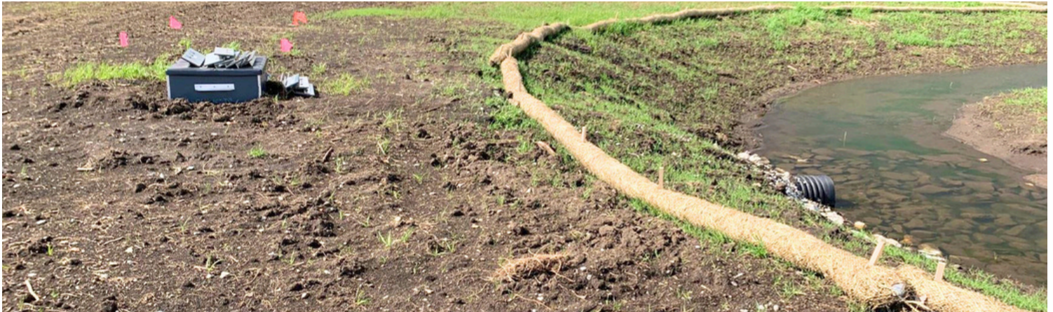
Photo: Water control box next to newly restored oxbow. The water control box can regulate tile flow into the oxbow.
