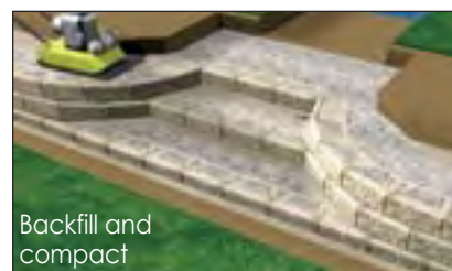
Install wall out from stairs
