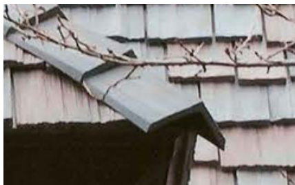
Hip Cap with Corner Overhang
