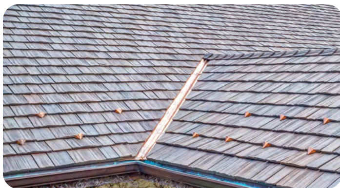
Figure 3.6.6 Open Valley Example with minimum 1" center crimp
