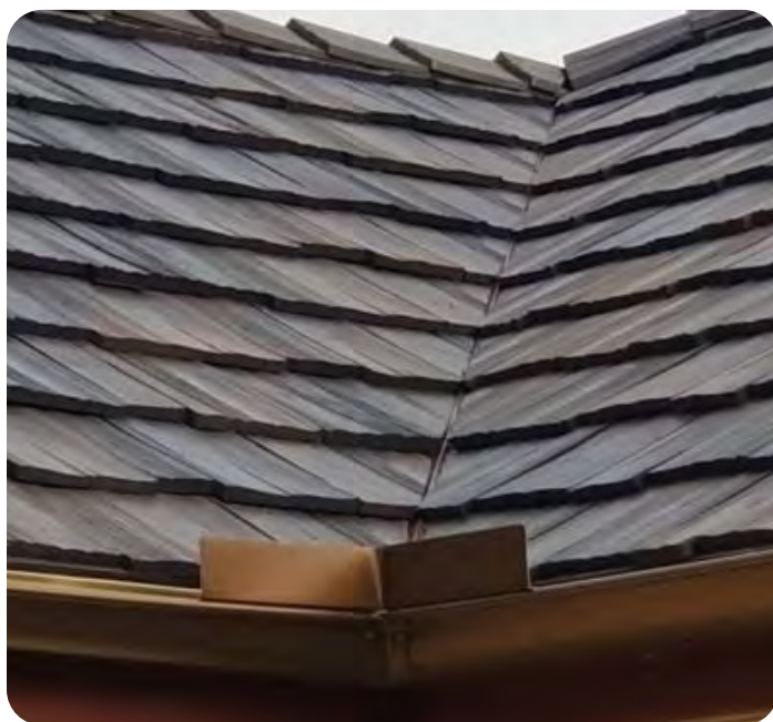
Figure 3.6.7 Closed valley example with 1 ½" center crimp
