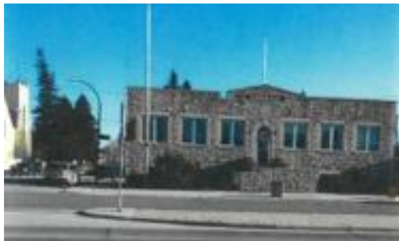
Collegiate and Portage, The Chapman Building, St. James Anglican in background
