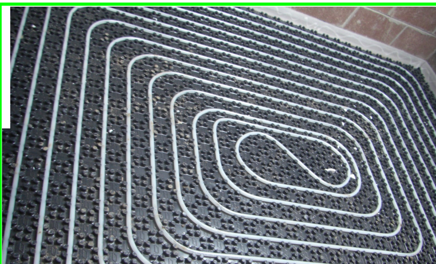
Insulation boards 1000 x 1000 mm with pipe fixings. Without insulation or insulation thickness 11 mm Overall thickness 29mm Centre to centre distance 50 mm or multiples
