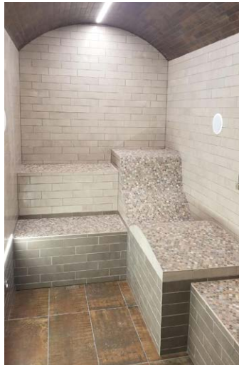
Custom shower benches created with HYDRO-BLOK 2" Building Board with dual Linear Drains and floor insulation for a Commercial Steam room project.
