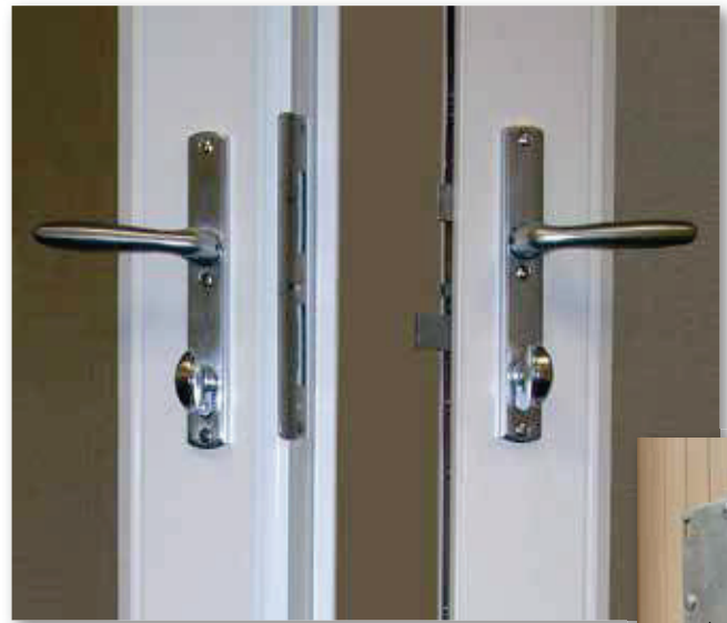
Heavy Duty Steel Plate Reinforces jamb against break-in force.
