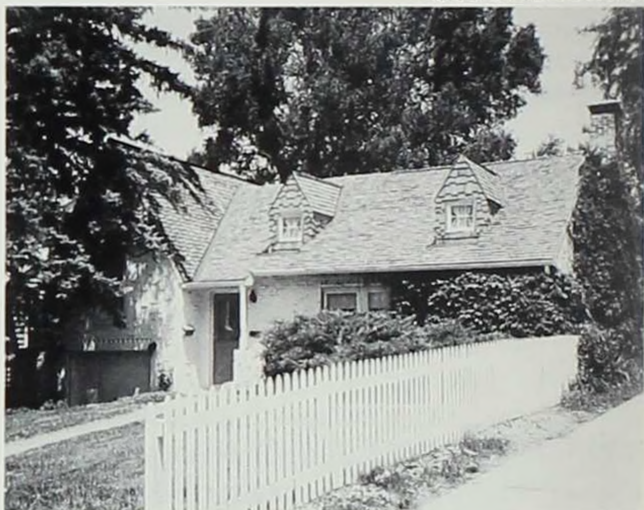
Here, Moffitt laid shingles in a thatch pattern, and used the ends of bricks for texture, window, and garage trim.
