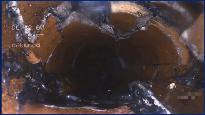
Major pipe damage found between 10-18 feet upstream from driveway manhole. Repair required
