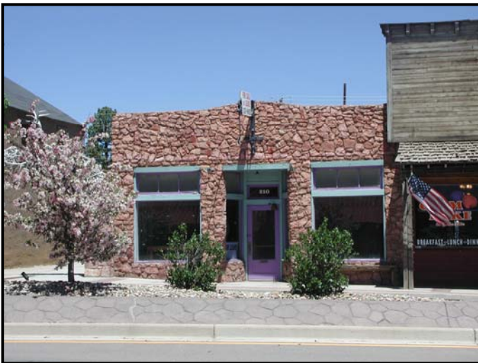
Old Post Office, 210 West Midland Avenue, 5TL3455, 1937.
