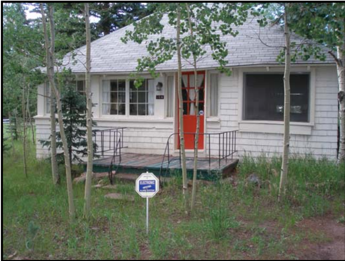
Sonnen Cabin, 106 East Bowman Avenue, 5TL3477, 1928.
