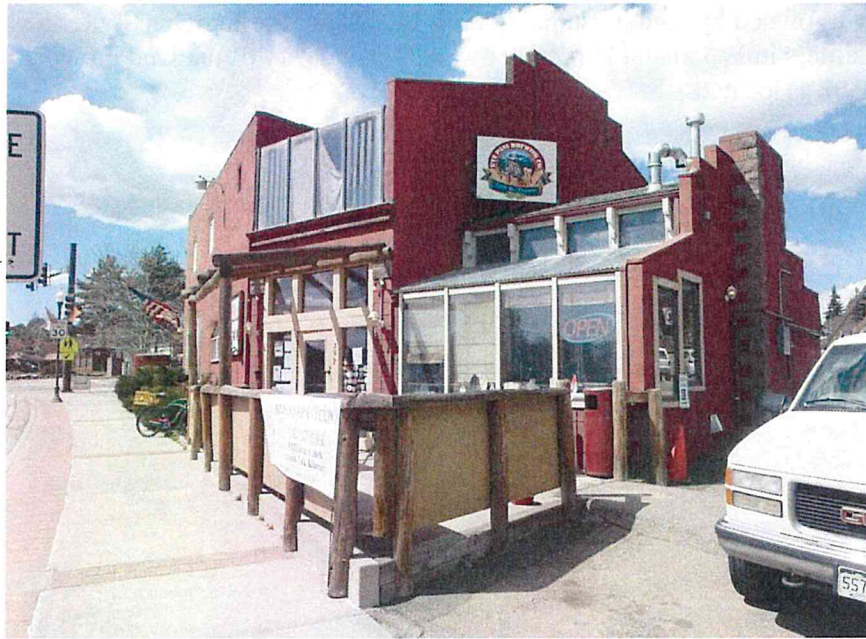
Figure 5-4: View of commercial building 5TL.4149. Looking west-northwest.
