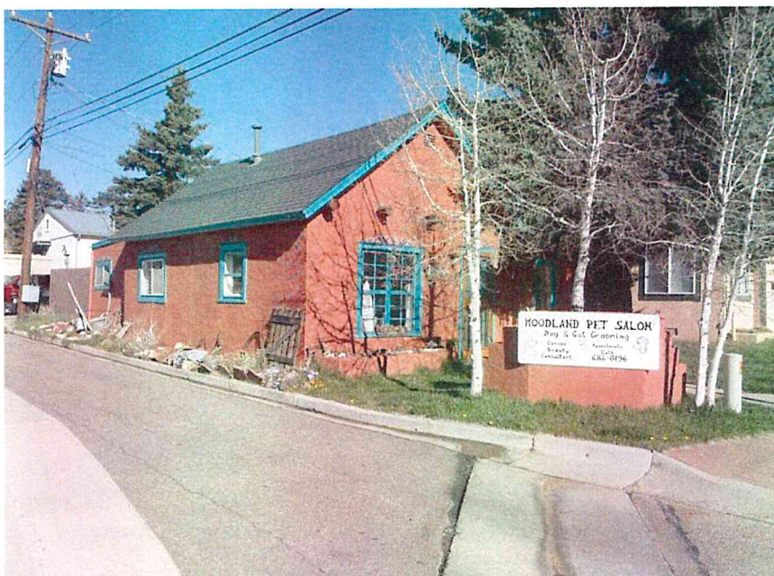
Figure 5-8: View of converted residence 5TL.4153. Looking northwest.
