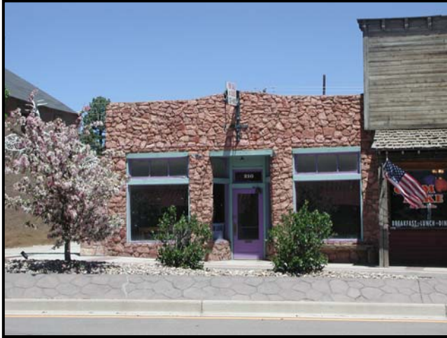
Old Post Office, 210 West Midland Avenue, 5TL3455, 1937.
