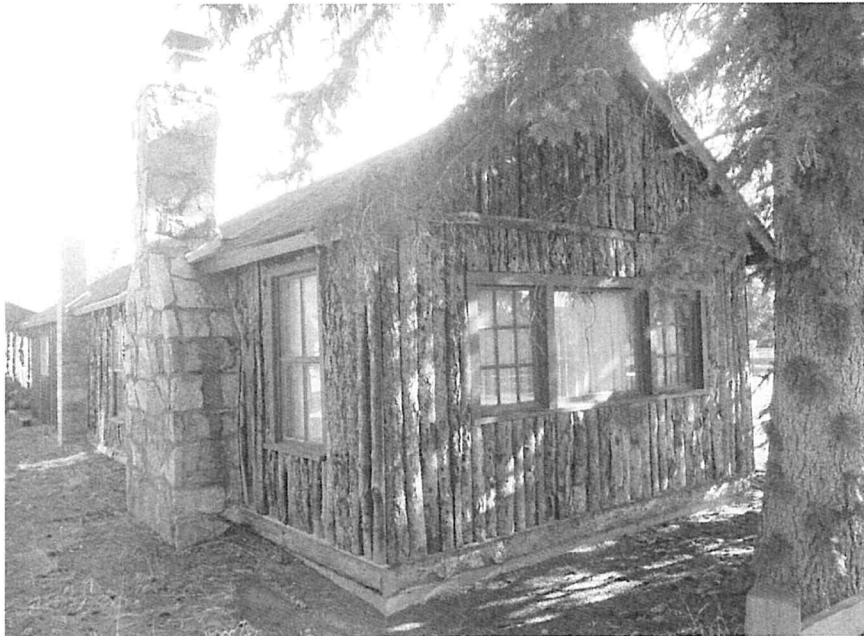
Figure 5-22: View of residence 5TL.4166. Looking northeast.
