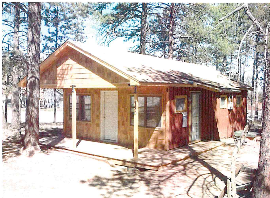
Figure 5-15: View of residence 5TL.4160. Looking northwest.
