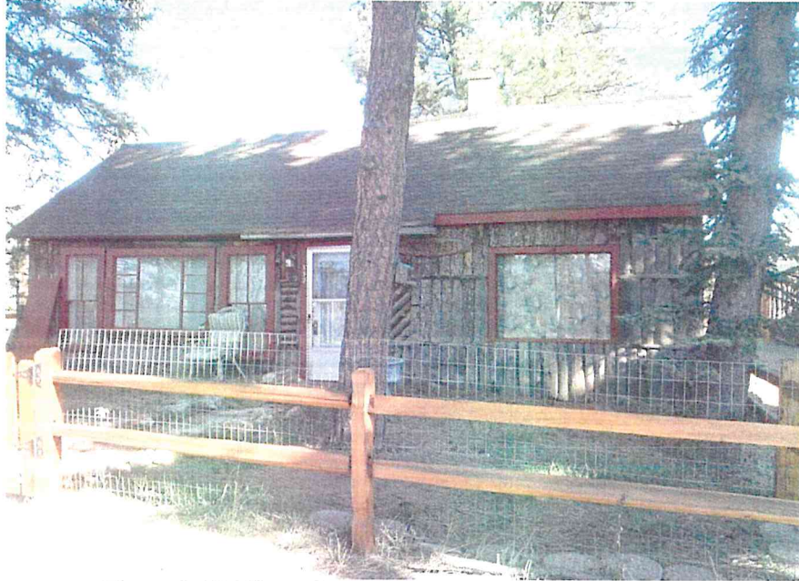
Figure 5-17: View of residence 5TL.4161. Looking north.
