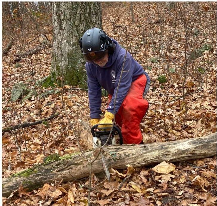
by Wayne Limberg: Jim Fetig cuts a blowdown for use as a check dam.
