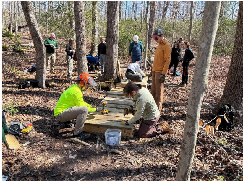
Photo by Dennis Calhoun: Justin Loyd and Amy Stulman fastening the foot boards
