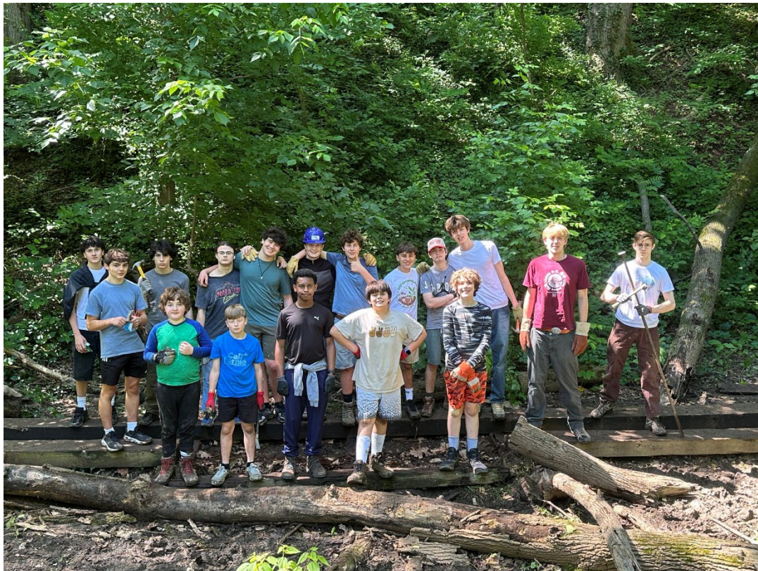
Troop 33 Scouts Having Completed Demolition of Boardwalk
