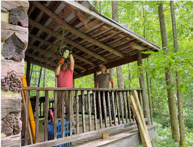
by Nick Green: Lee Howard and Noah Green begin demolition
