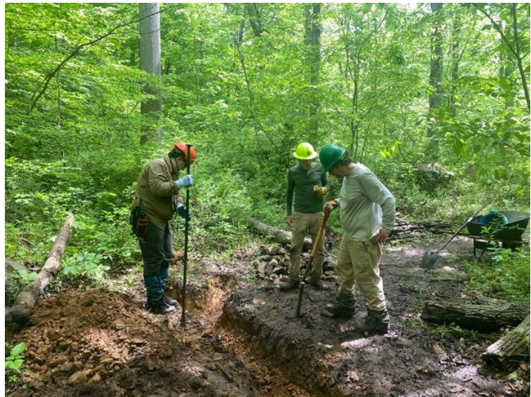
Tori Wenig, Jeff Clyman, and Jim Tomlin dig the French drain
