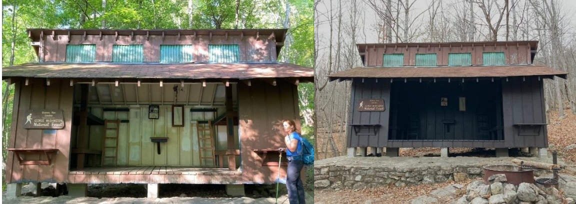
Boones Run Shelter Before and In-Progress Painting
