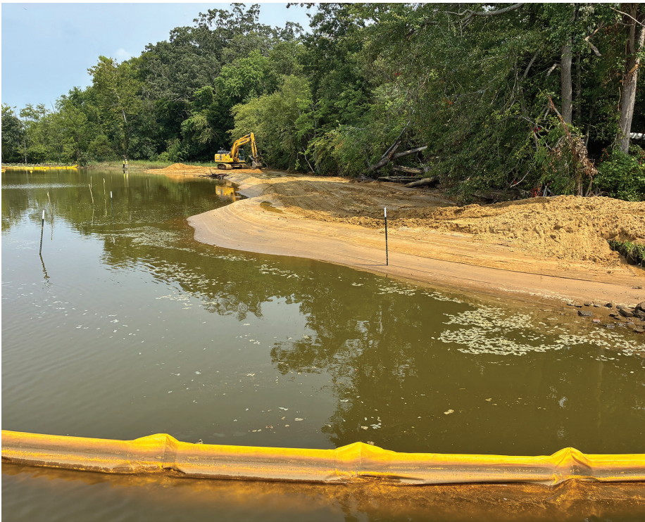
Filling material being delivered and distributed at the shoreline restoration site by Environmental Quality Resources, L.L.C.
