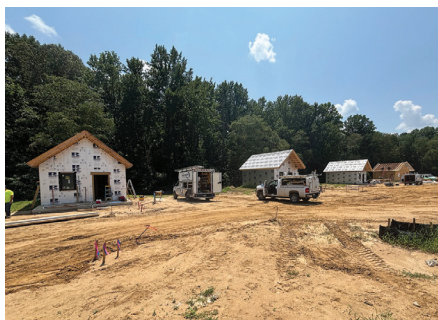
A lot of hard work went into building the JBERD cabins.
