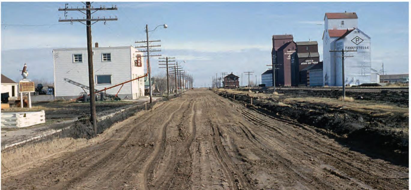
1961-08-00 Fannystelle, MB: Main Street under construction. Paving the streets of town.
