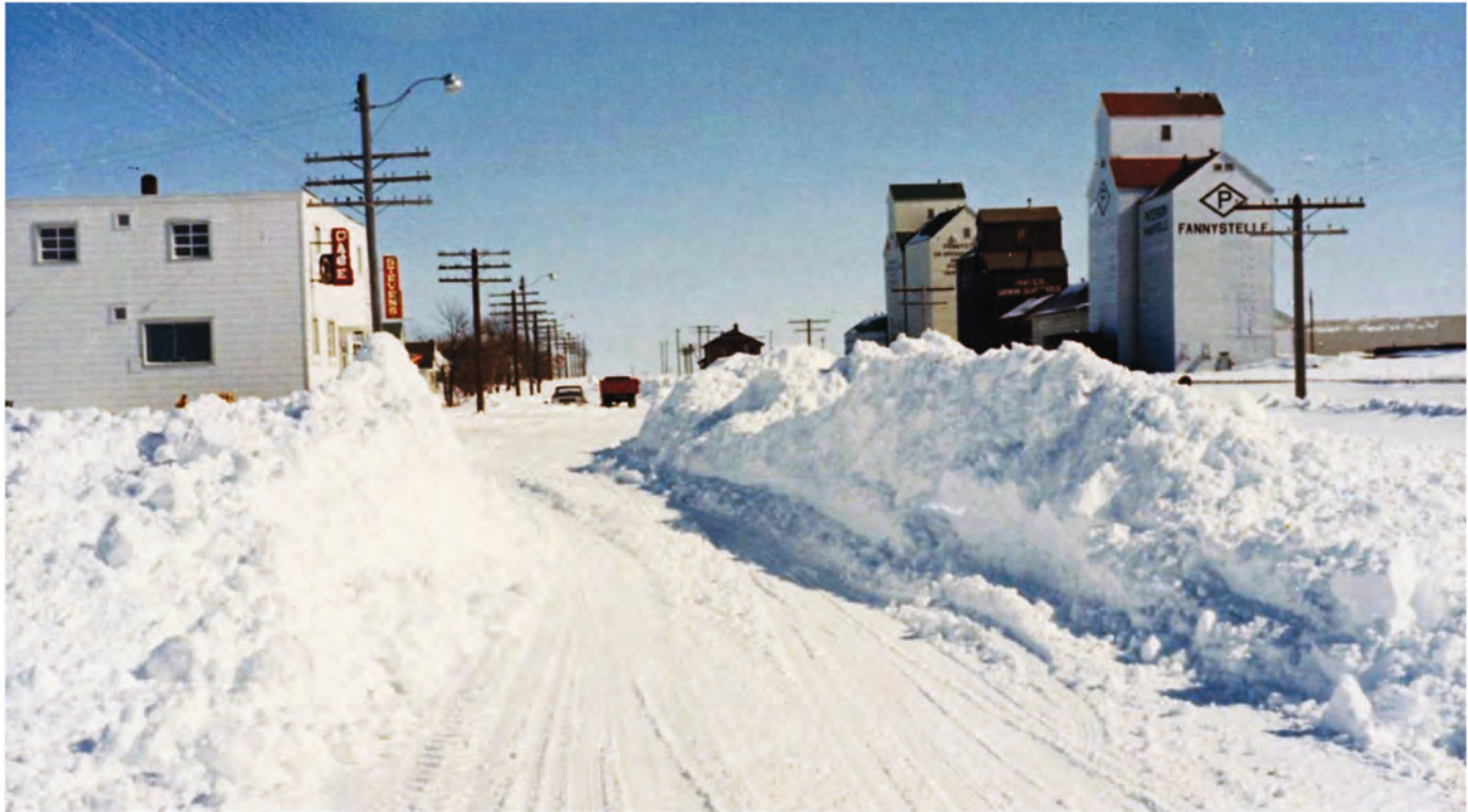
1966-03-27: Fannystelle – View looking east with Stevens Lumber Ltd.
