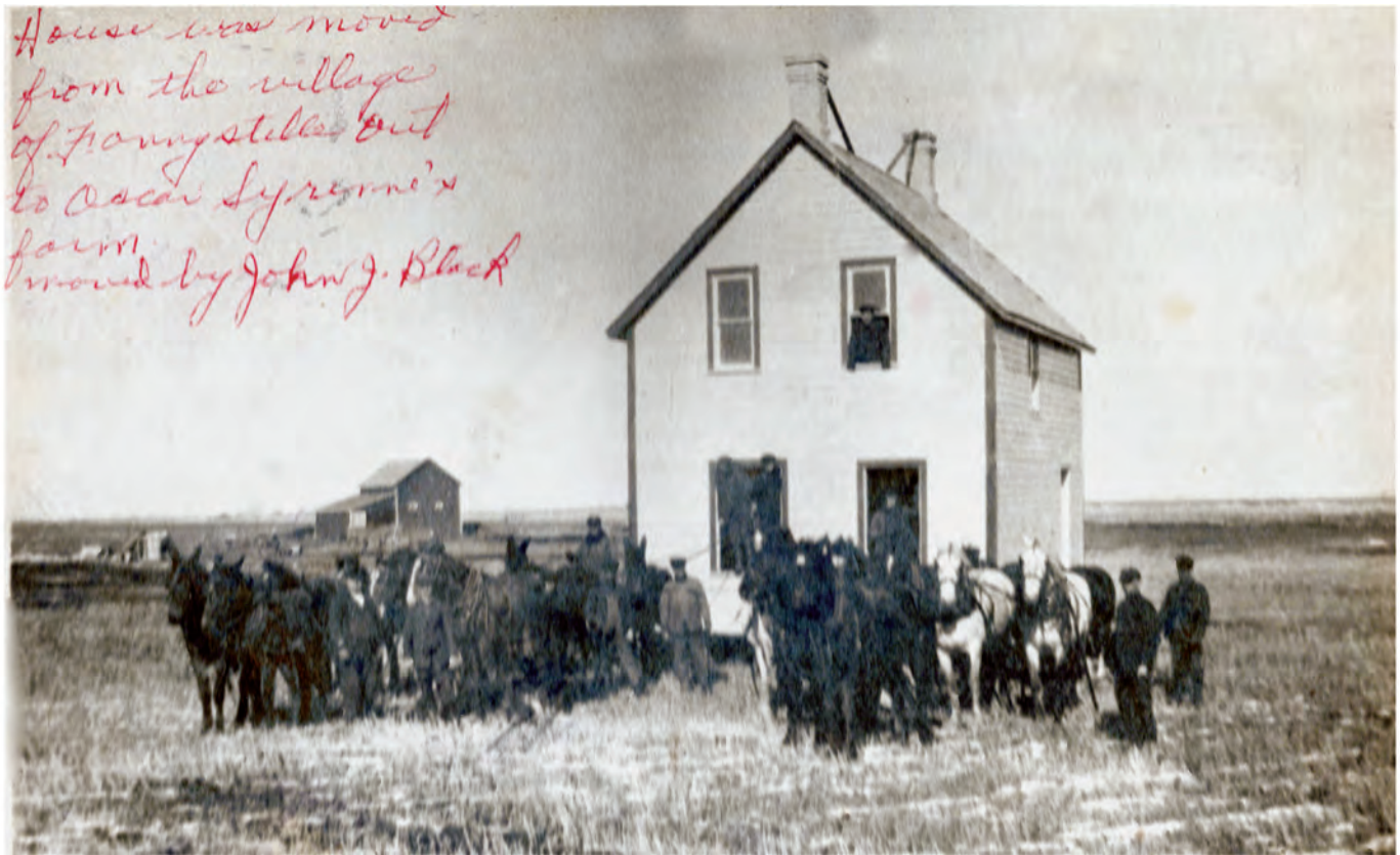
1920-03-00: Work party moving Oscar Syrenne's house using horses. The house on skids was dragged on frozen ground from Fannystelle to the Syrenne farm. Mover: John J. Black, the local blacksmith.
