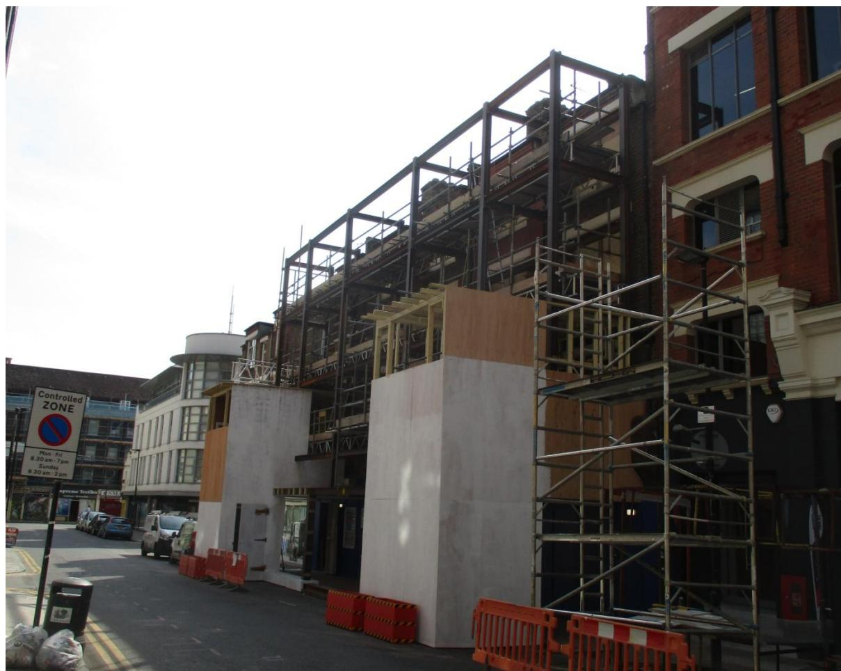
Once both temporary structures were built and tied together, they then remained as a stable support for the rest of the reconstruction project for the further 15 months.
