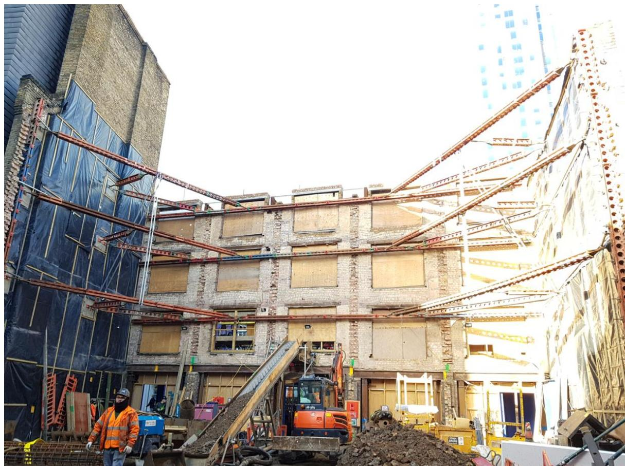
When the work started and the existing building behind the facade was demolished, the main contractor then required further space for his temporary storage of material as well as workmen welfare facilities. MSJs instruction was quickly expanded so to create a further temporary structure on the roadside of the by now retained facade, and which was then created as a set of steel frames connected to the already built facade retention wall beams.
