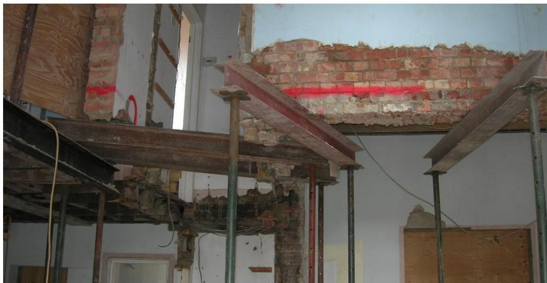
Regarding the temporary works, this can take a shape of the traditional beam and needle arrangement, or in the case of lighter structures what is customarily known as a strong boy.
