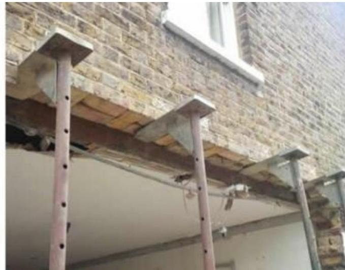
Sometimes these temporary works are requested to be carried out from one side of the subject will only, so not to damage the internally finished surfaces. An example is shown on the photo below.
