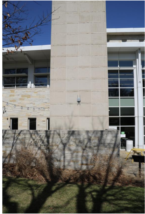
View of Patio Wall from
