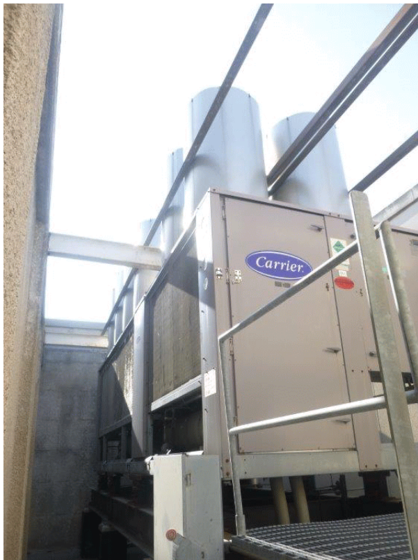
Air Cooled Water Chiller
