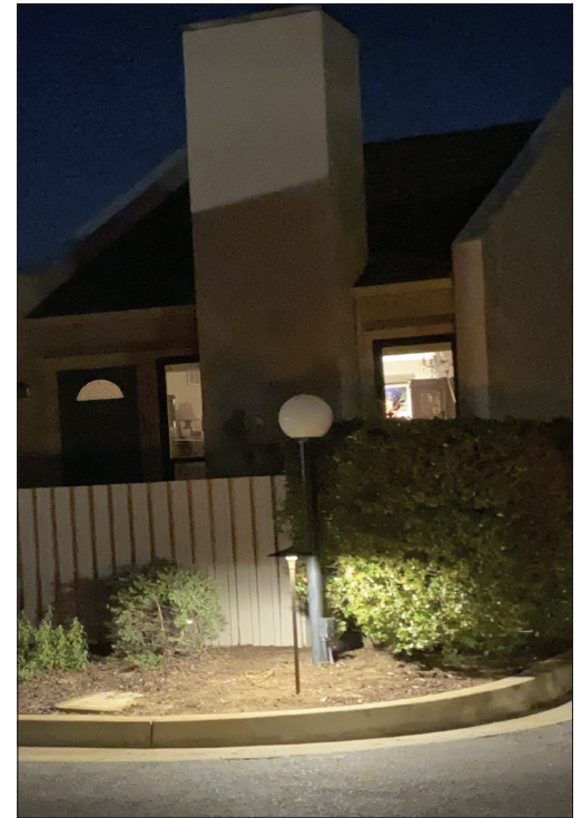
Old pole (in background) spread glare. New one focuses light only where needed.
