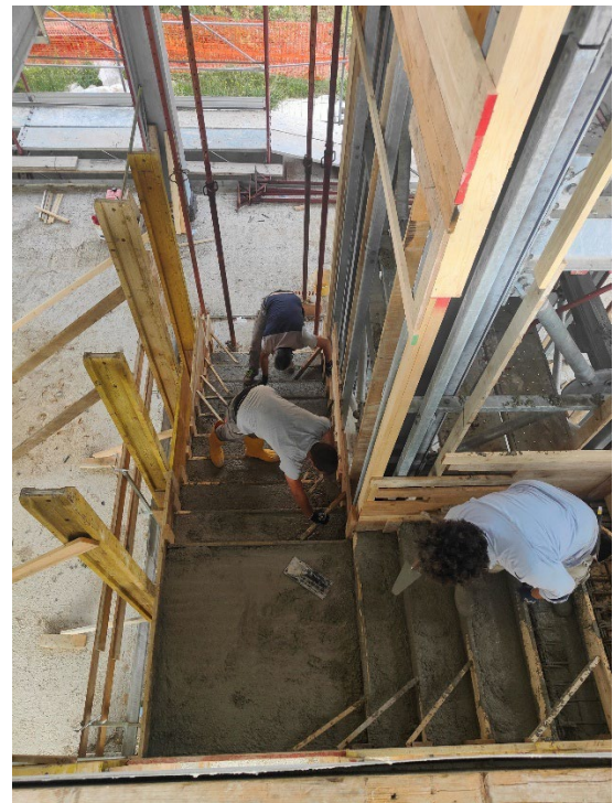
Figure 6.38: Concrete casting of staircase
