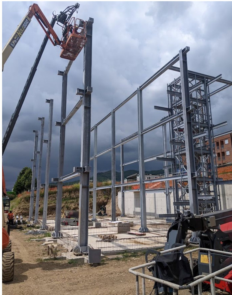
Figure 6.20: Erection of steel beams
