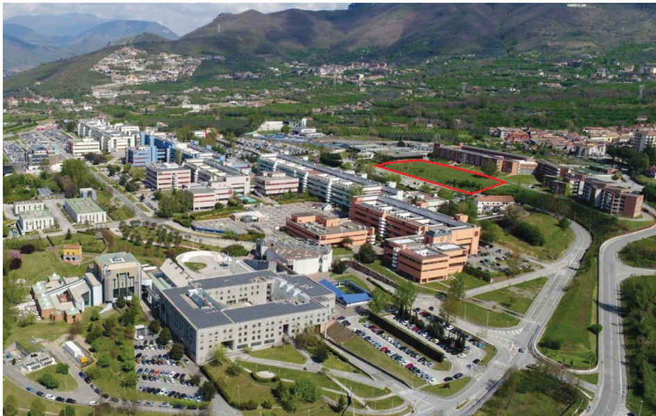
Figure 1.1: Main Campus of Salerno University with the construction site
