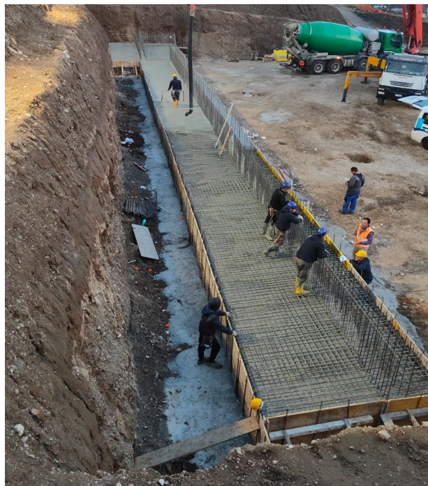
Figure 6.6: Concrete casting of restraining wall
