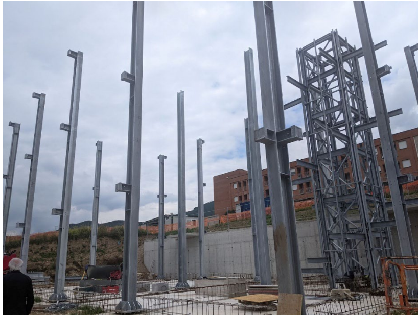
Figure 6.19: Erection of steel columns
