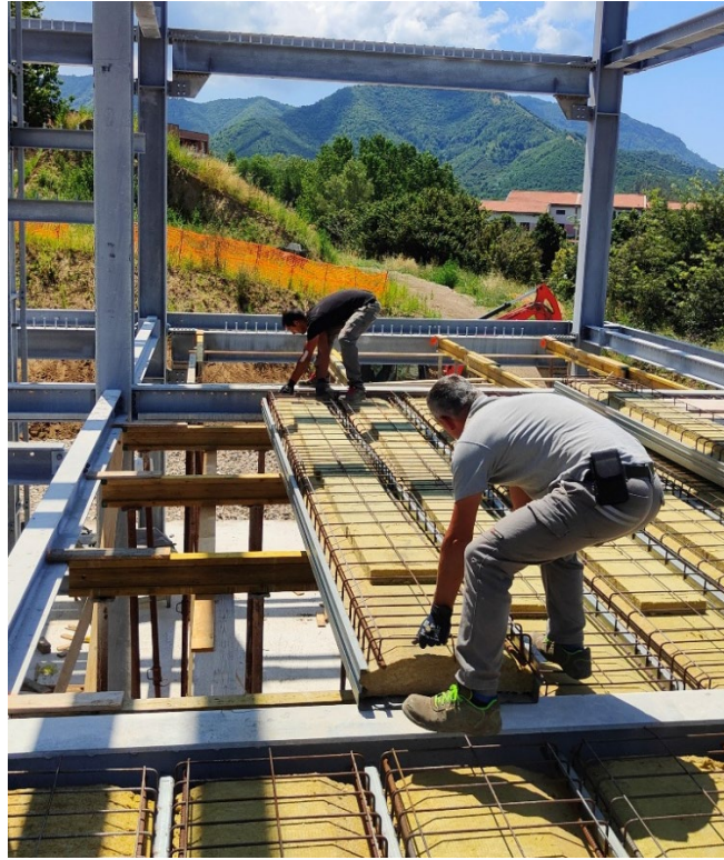
Figure 6.27: Assembly of Cofradal panels for first floor
