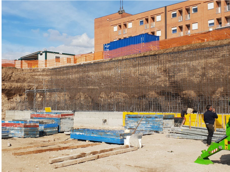
Figure 6.7: Positioning of rebars of the retaining wall
