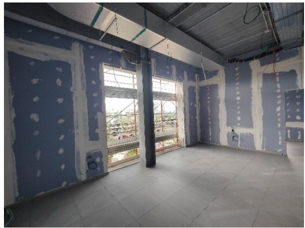
Figure 6.40: Installation external and internal partition walls
