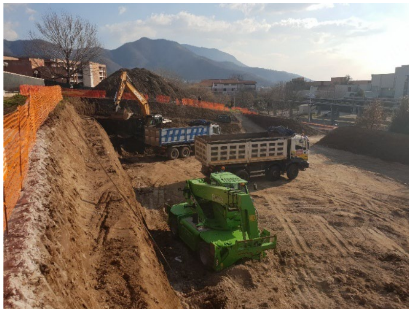
Figure 6.4: Ground stored near the construction site
