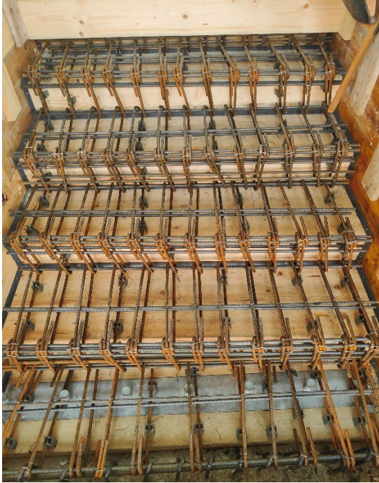
Figure 6.37: Staircase reinforcements
