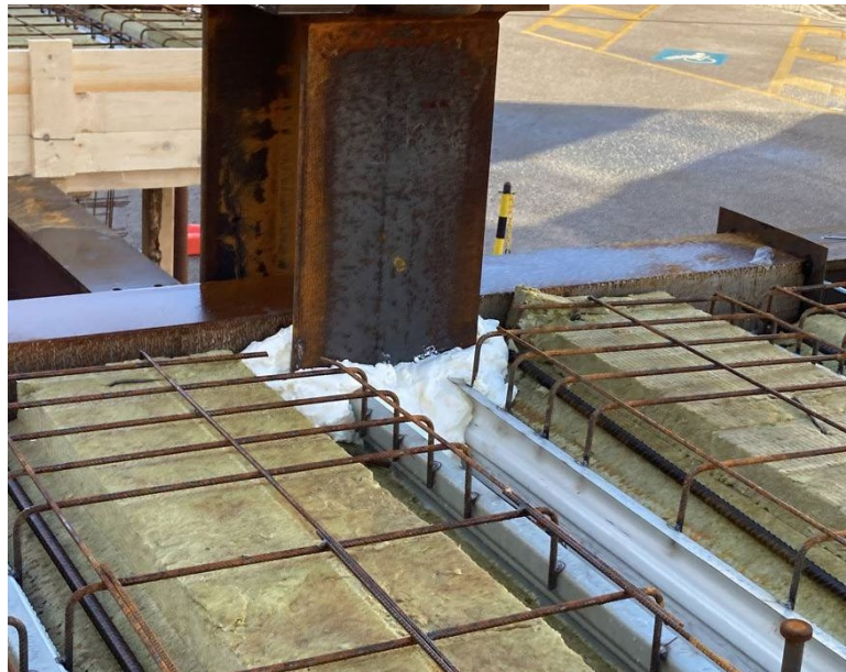
Figure 3.11: Disconnection detail in the joint area
