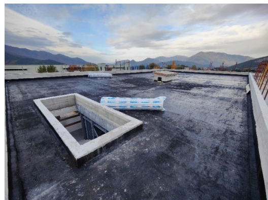
Figure 6.36: Thermal insulation and waterproofing of third floor
