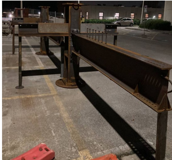
Figure 3.8: Specimen before placement of Cofradal
