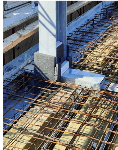
CONNECTION REALIZED IN SITU
