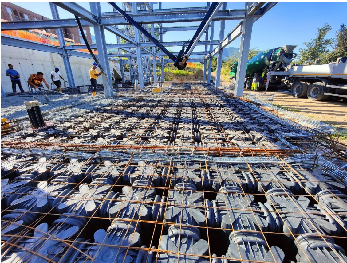
Figure 6.26: Concrete casting of upper part of the foundation and of the crawl space
