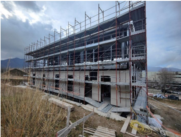
Figure 6.40: Installation external and internal partition walls
