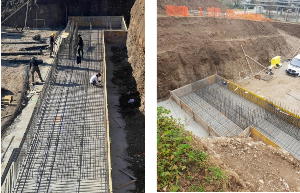
Figure 6.5: Positioning of the rebar for the foundation
