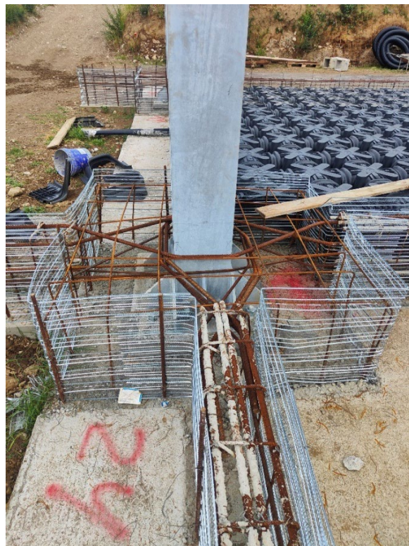
Figure 6.24: Positioning of the Iglù formwork
