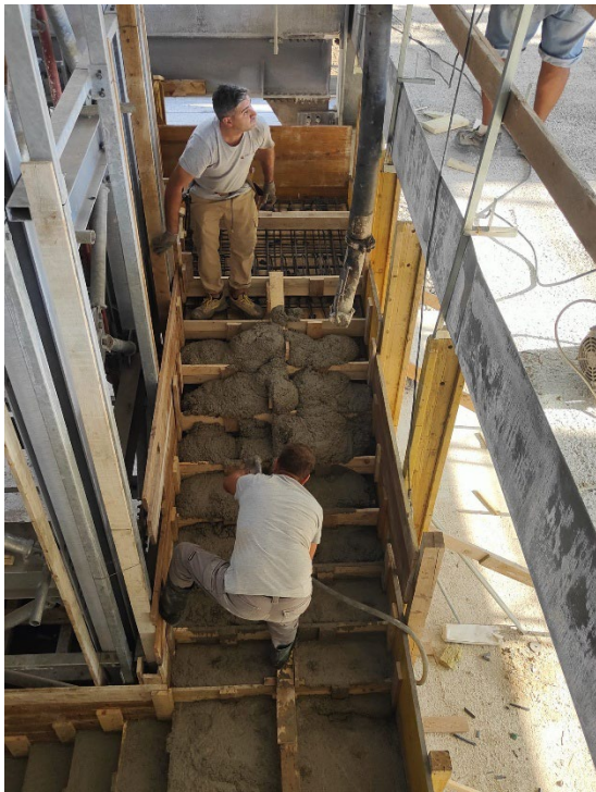
Figure 6.38: Concrete casting of staircase
