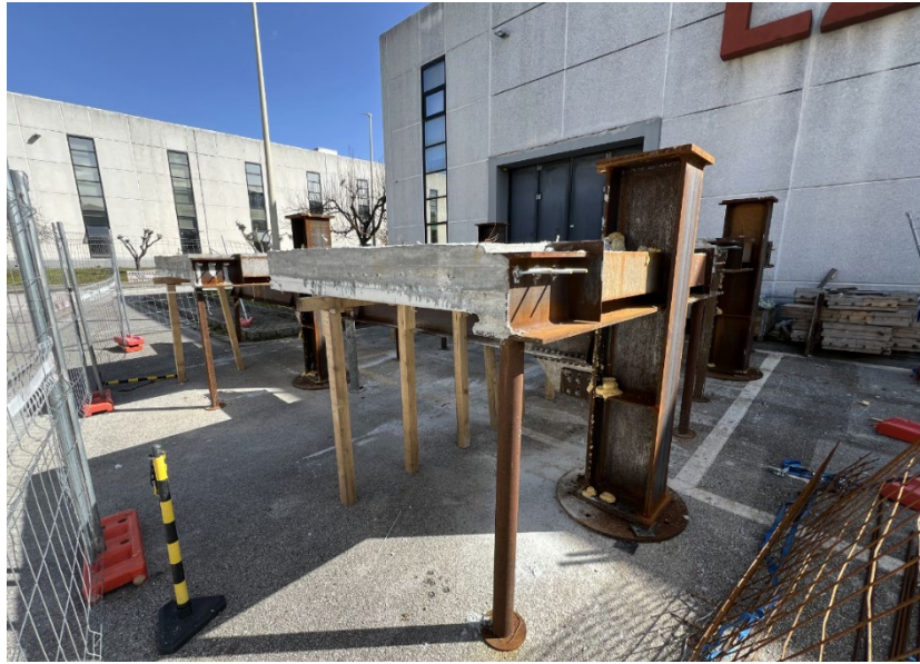
Figure 3.10: Specimen after the curing of concrete
