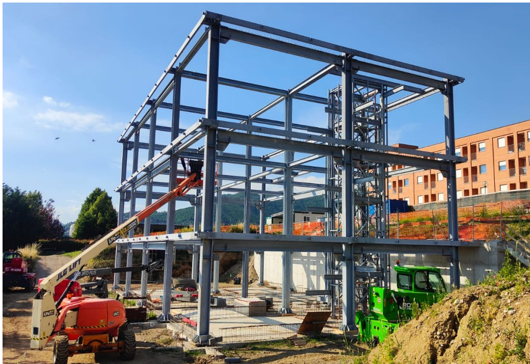
Figure 6.22: Erection of steel beam equipped with Freedom connections
