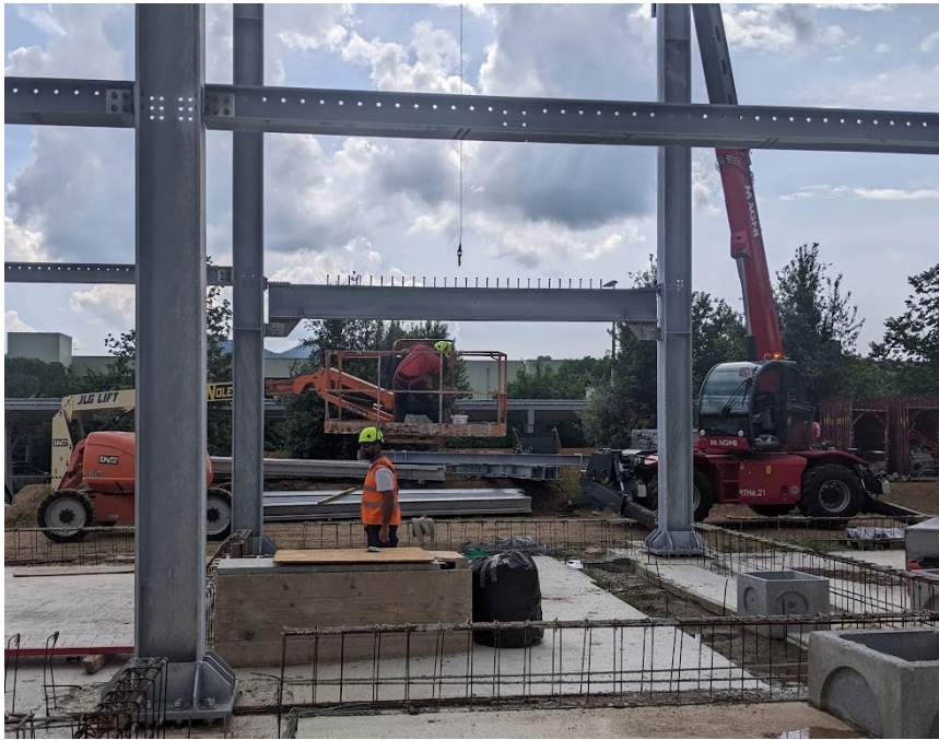
Figure 6.21: Erection of first steel beam equipped with Freedom connections
