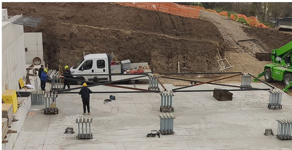
Figure 6.10: Positioning of the base plates and anchor bolts of the steel columns
