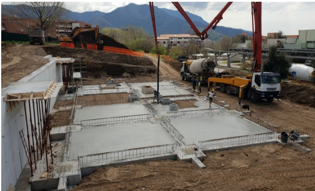
Figure 6.18: Realization of the concrete slab constituting the base for the iglù formwork
