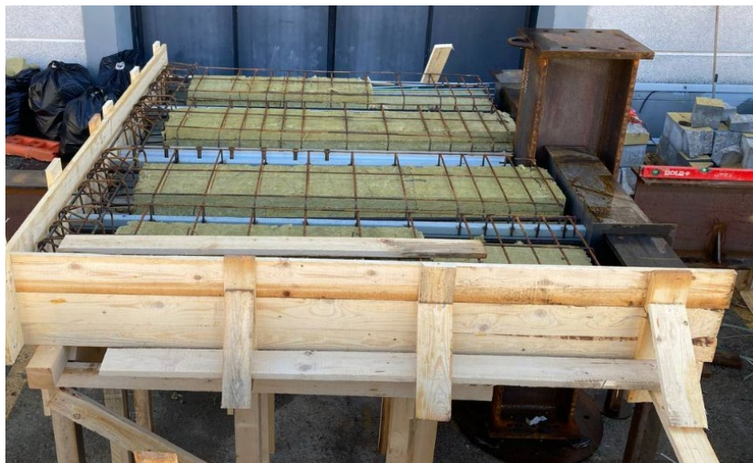
Figure 3.9: Specimen after placement of Cofradal
