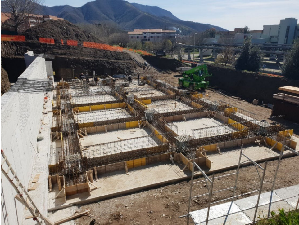
Figure 6.13: Foundation reinforcement
