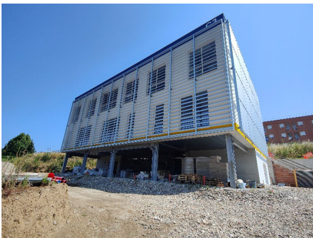
Figure 6.43: Installation of the external sunshades
