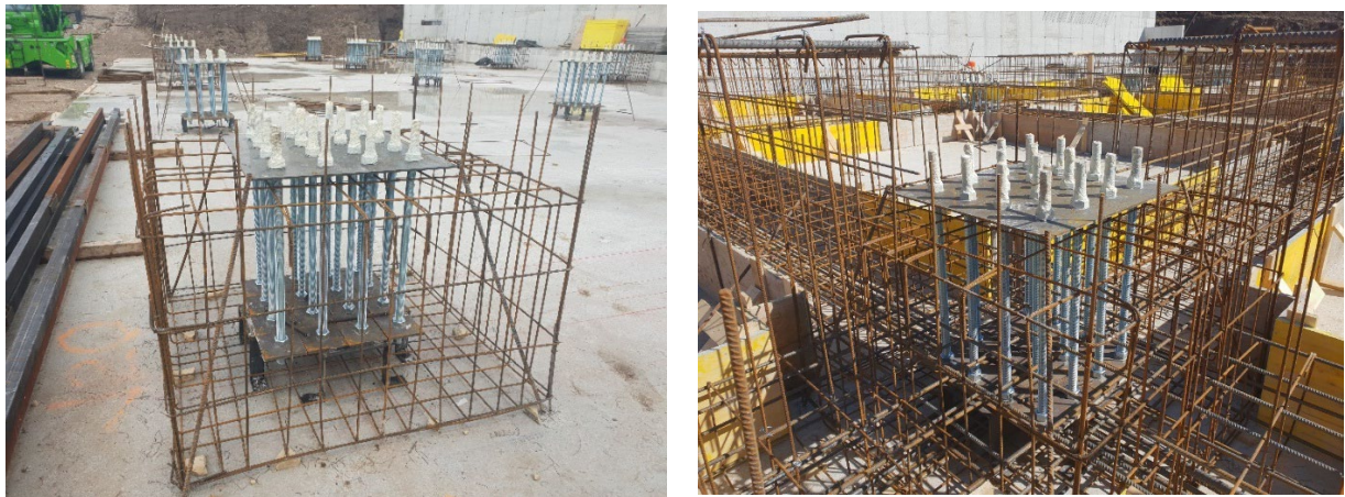
Figure 6.12: Foundation reinforcement
