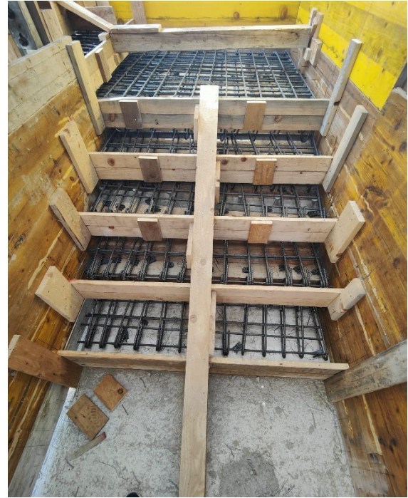
Figure 6.37: Staircase reinforcements
