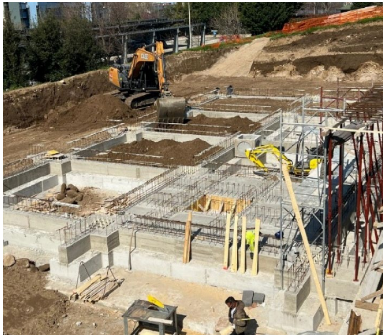
Figure 6.16: Filling of the spaces between the foundation beams with the soil coming from the excavation phase
