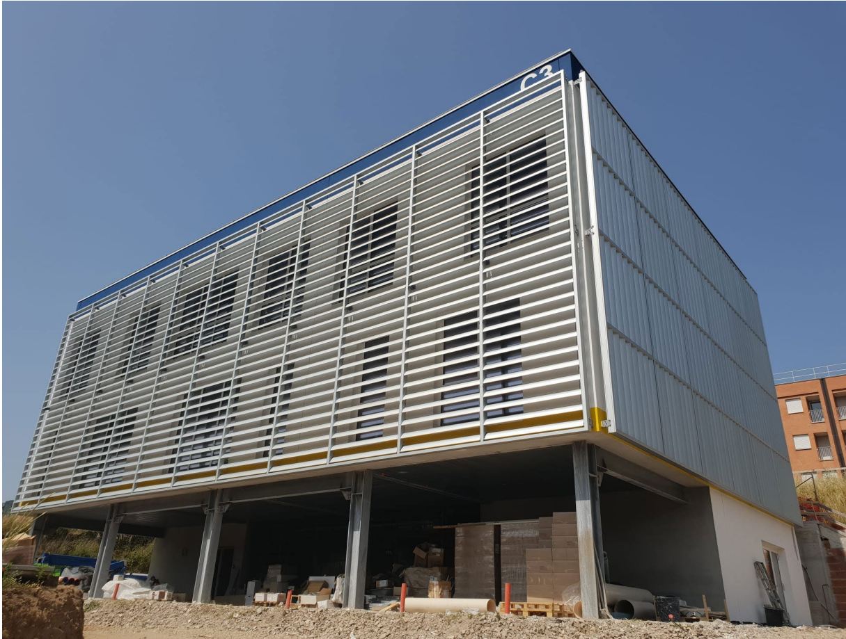
Figure 1.21: Final appearance of the façade of the building under construction (June 2025)
