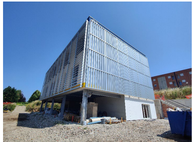
Figure 6.43: Installation of the external sunshades
