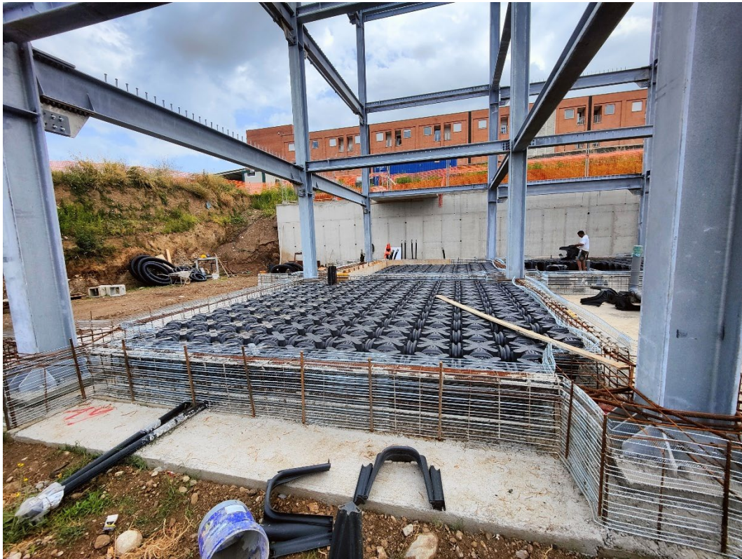
Figure 6.25: Positioning of the Iglù formwork
