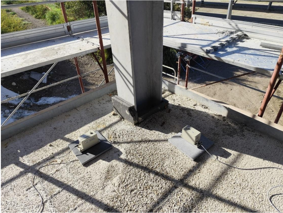
Figure 3. Sensors 30H and 35H in the lower right corner of the building with reference to Figure 1
