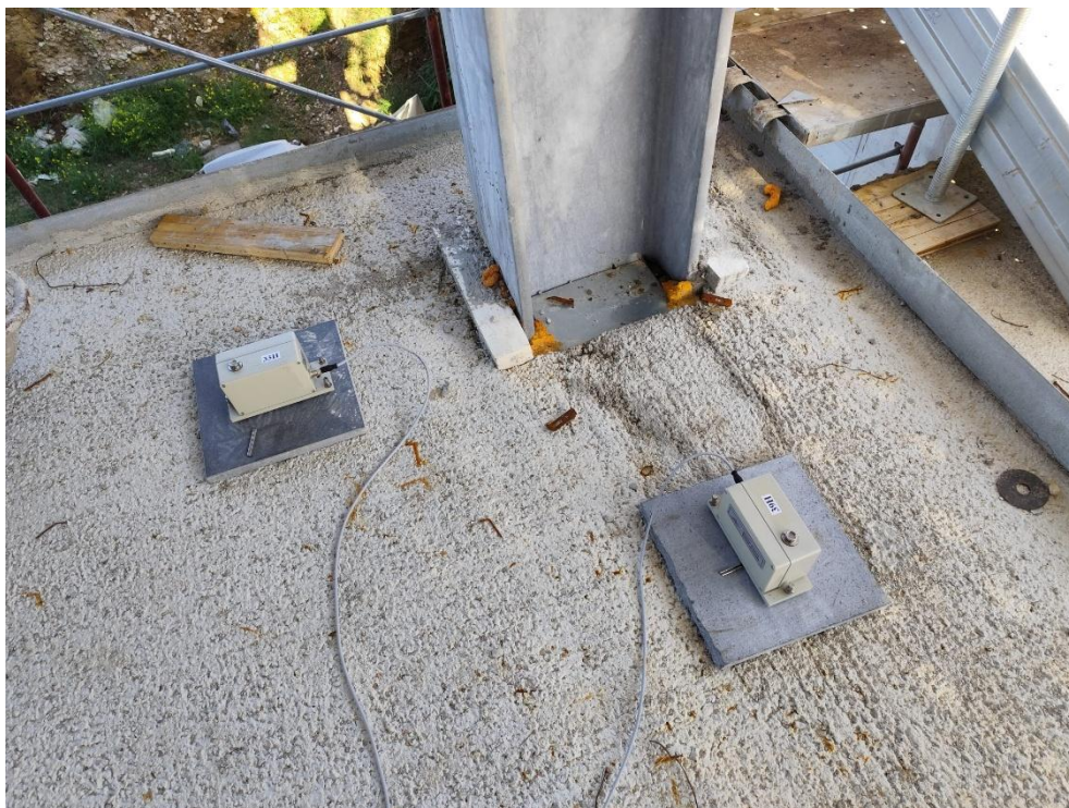
Figure 2. Sensors 33H and 39H in the lower right corner of the building with reference to Figure 1
