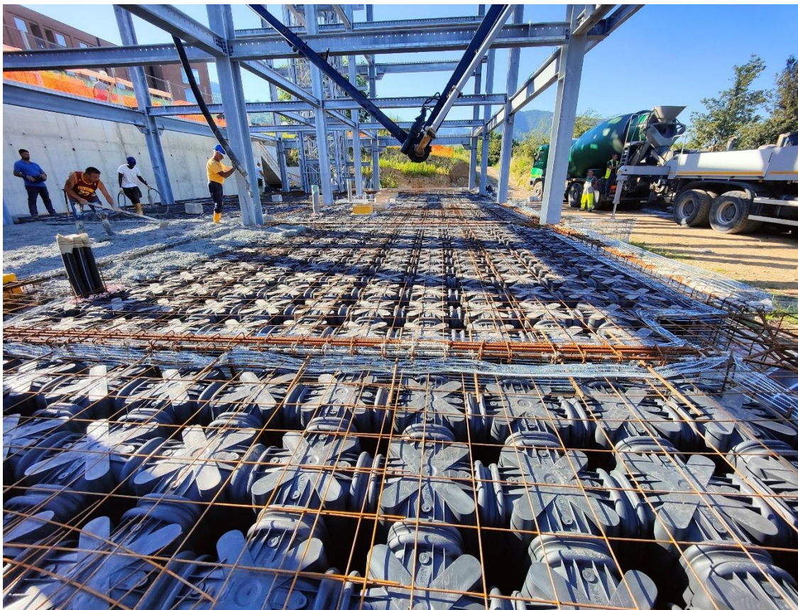
Figure 6.26 – Concrete casting of upper part of the foundation and of the crawl space
