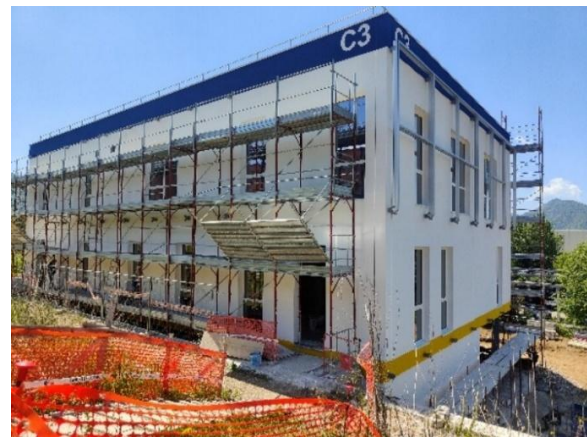
Figure 6.42 Installation of the suspended ceiling and painting of the interior and exterior walls
