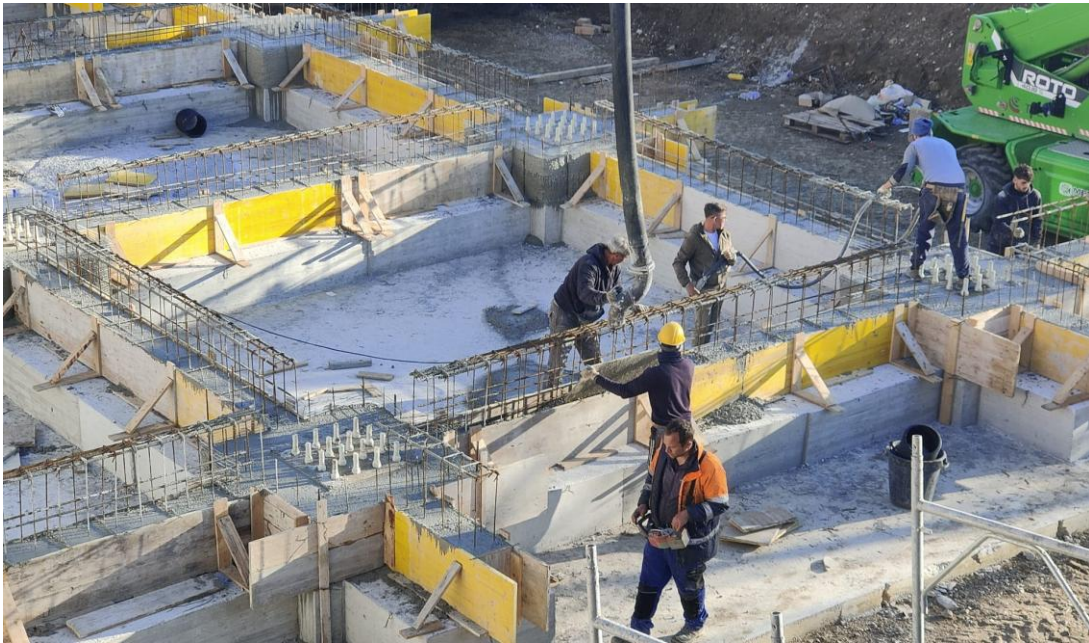
Figure 6.15 – Concrete casting of the upper part of the inverted foundation beams
