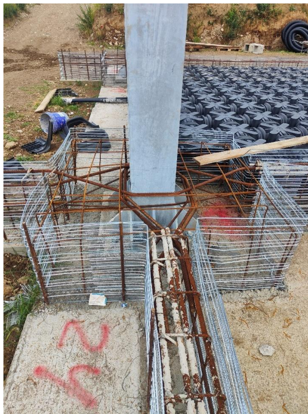
Figure 6.24 – Positioning of the Iglù formwork
