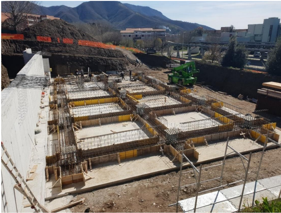
Figure 6.13 – Foundation reinforcement
