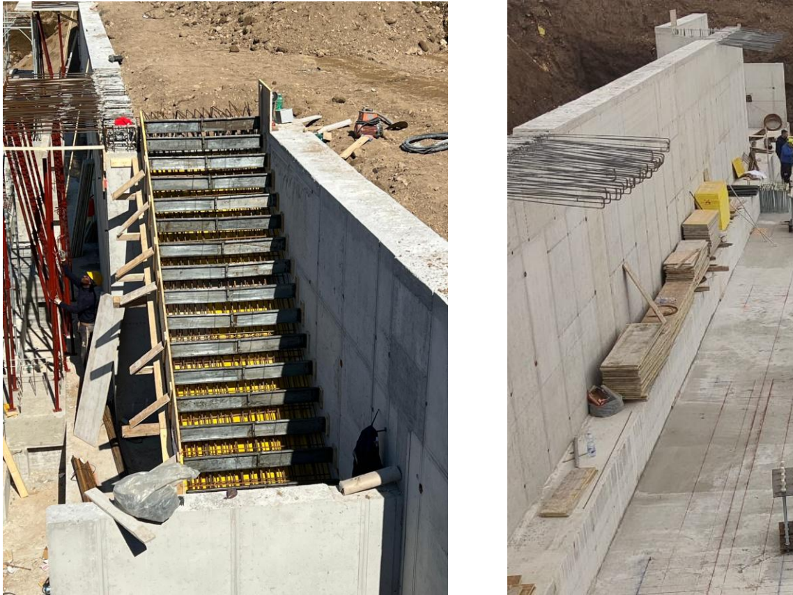
Figure 6.9 – Staircase and cantilever slabs realized on the retaining wall
