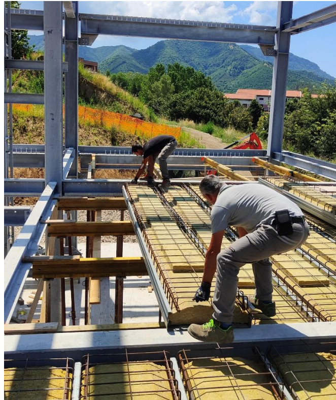
Figure 6.27 – Assembly of Cofradal panels for first floor
