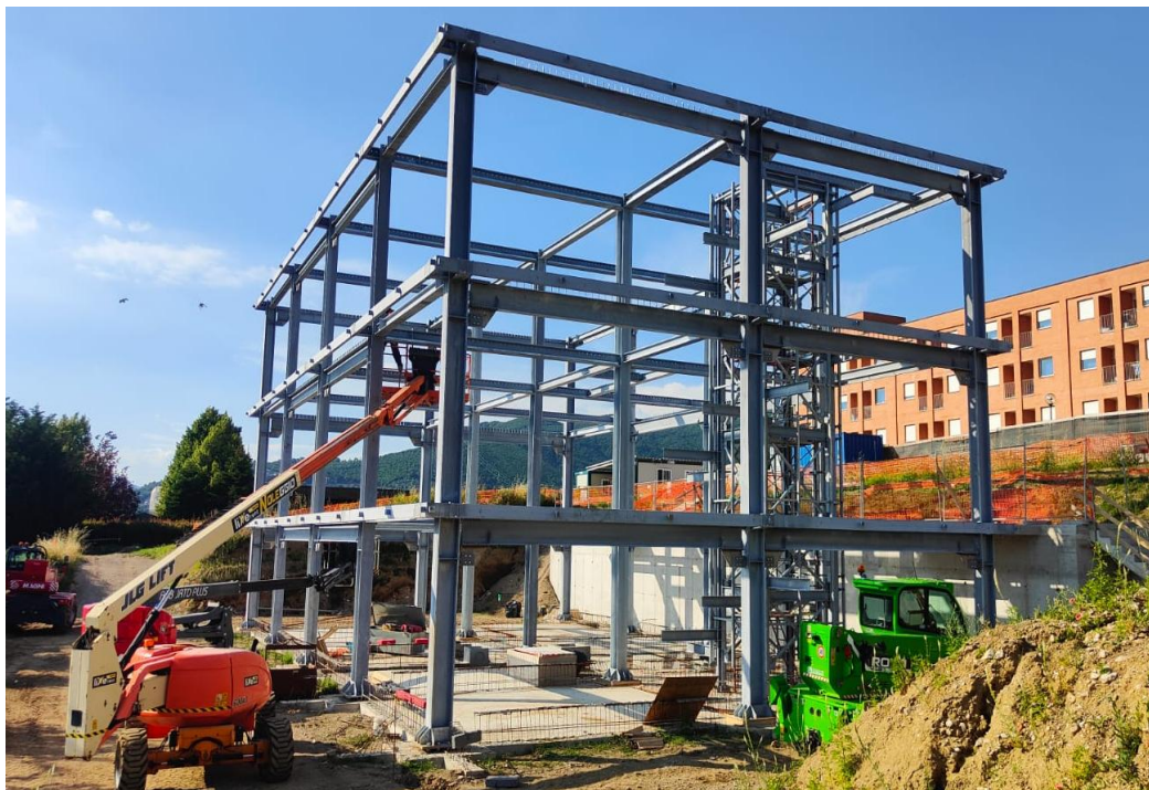
Figure 6.22 – Erection of first steel beam equipped with Freedom connections
