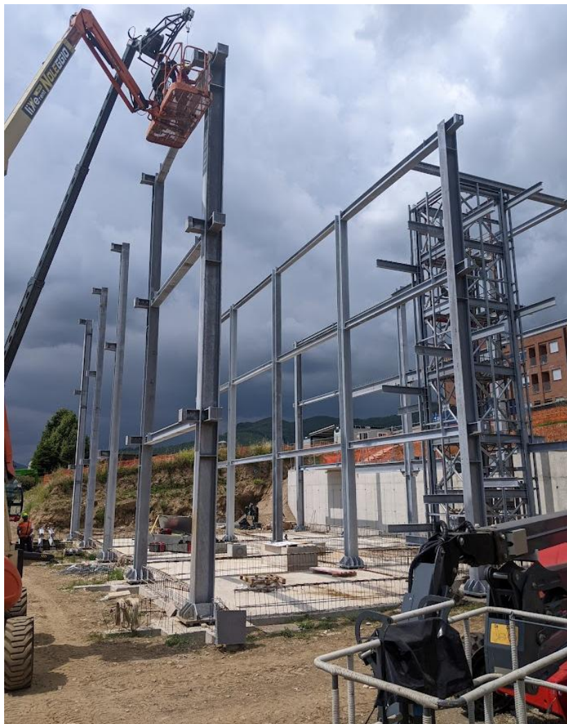
Figure 6.20 – Erection of steel beams
