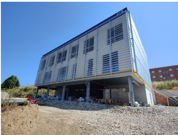
Figure 6.43 Installation of the external sunshades
