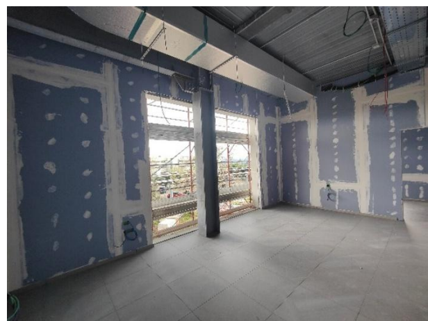
Figure 6.40 – Installation external and internal partition walls
