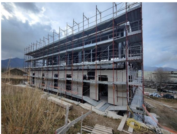
Figure 6.40 – Installation external and internal partition walls
