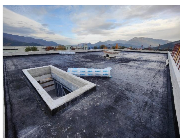
Figure 6.36 – Thermal insulation and waterproofing of third floor
