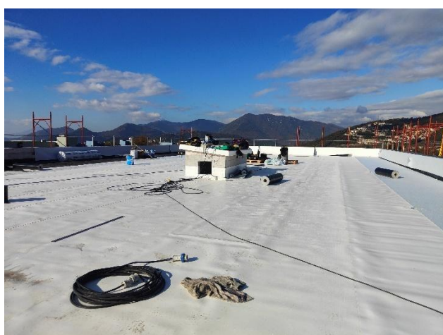
Figure 6.36 – Thermal insulation and waterproofing of third floor
