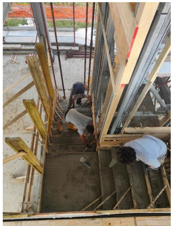
Figure 6.38 – Concrete casting of staircase
