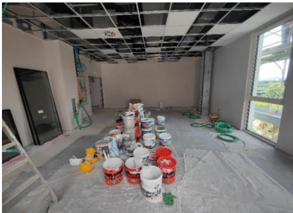
Figure 6.42 Installation of the suspended ceiling and painting of the interior and exterior walls
