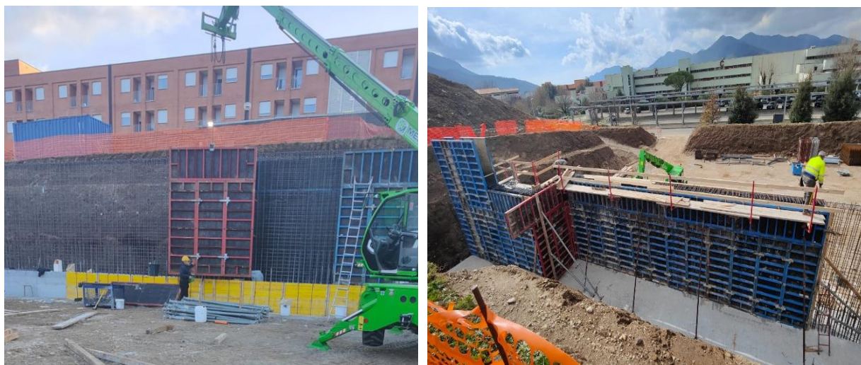
Figure 6.8 – Self-climbing formwork
