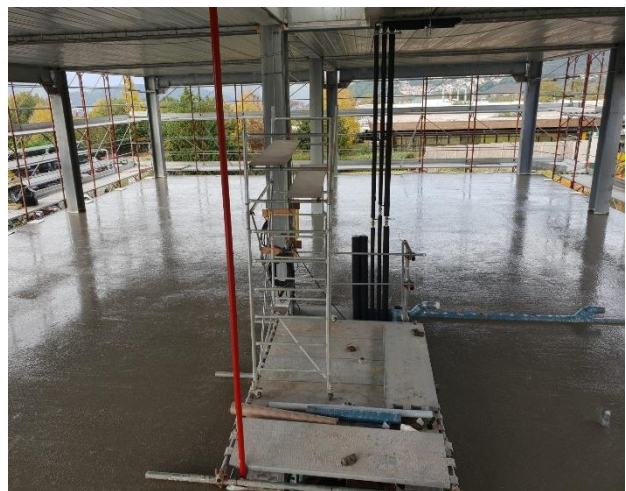
Figure 6.31 – Realization of the screed
