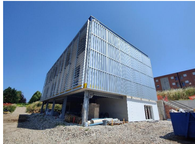
Figure 6.43 Installation of the external sunshades
