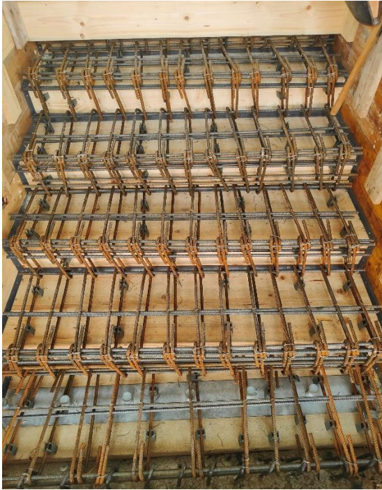
Figure 6.37 – Staircase reinforcements
