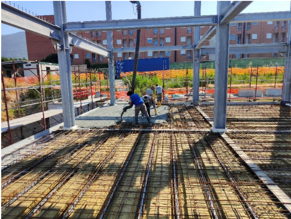
Figure 6.30 – Concrete casting of the first floor
