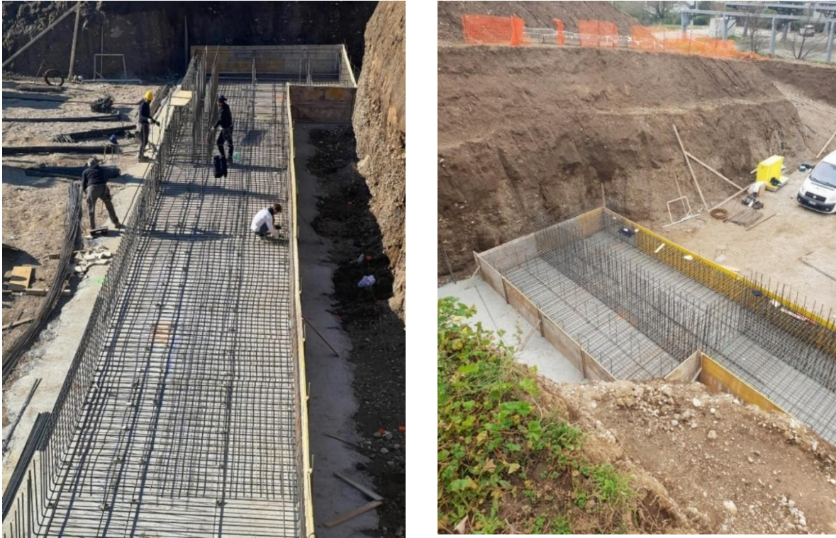
Figure 6.5 – Positioning of the rebars for the foundation
