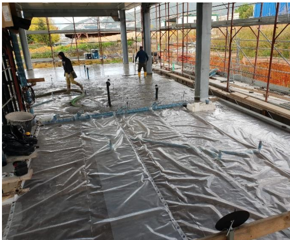
Figure 6.31 – Realization of the screed
