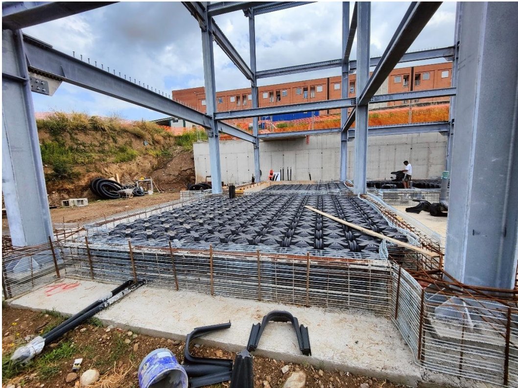
Figure 6.25 – Positioning of the Iglù formwork
