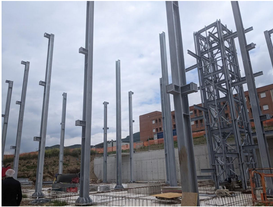
Figure 6.19 – Erection of steel columns
