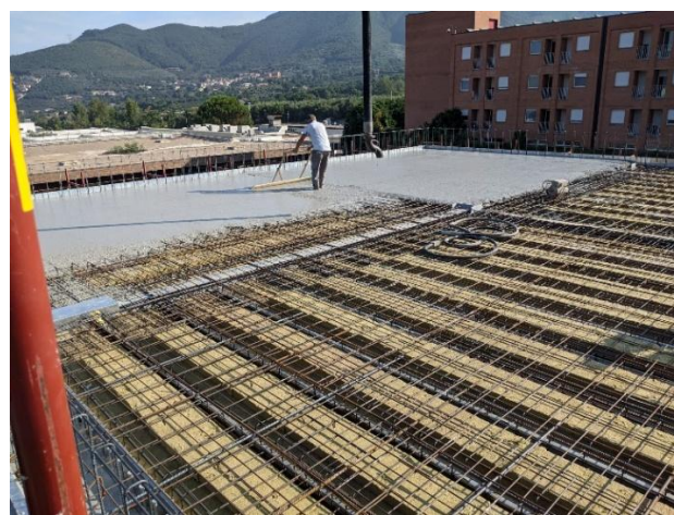
Figure 6.35 – Realization of third floor
