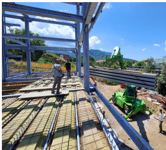
Figure 6.28 – Handling of Cofradal Panel from ground floor to first floor
