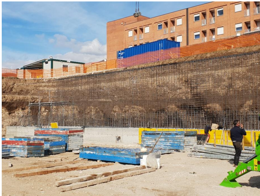
Figure 6.7 – Positioning of rebar of the retaining wall
