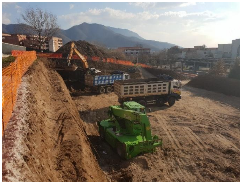
Figure 6.4 – Ground stored near the construction site
