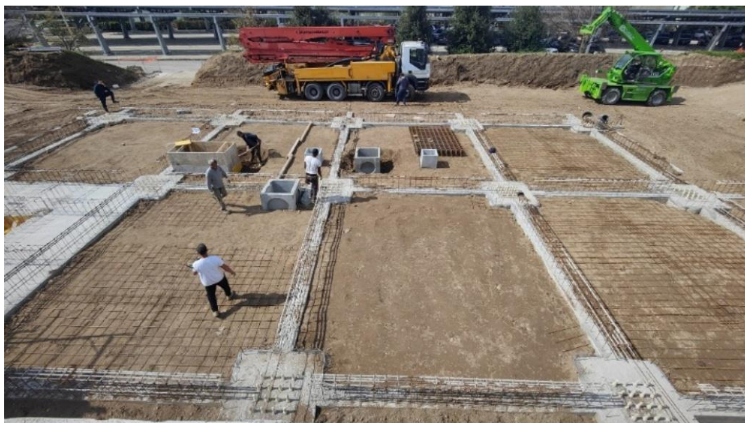
Figure 6.17 – Filling of the spaces between the foundation beams with the soil coming from the excavation phase
