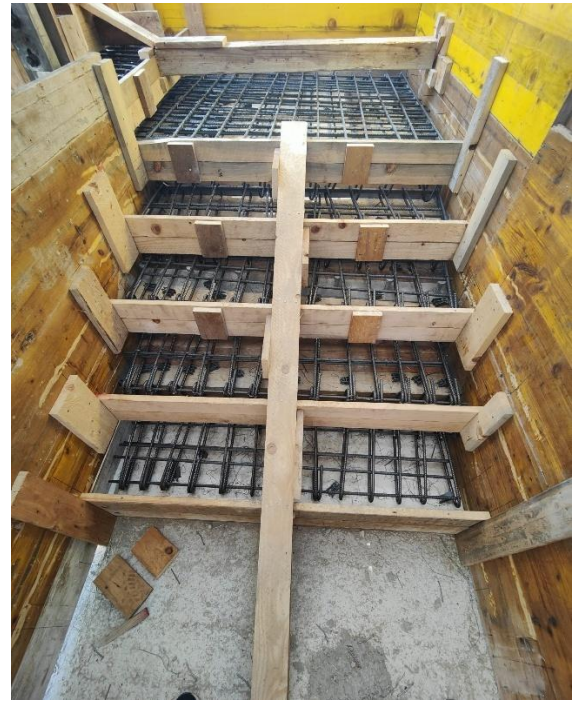
Figure 6.37 – Staircase reinforcements
