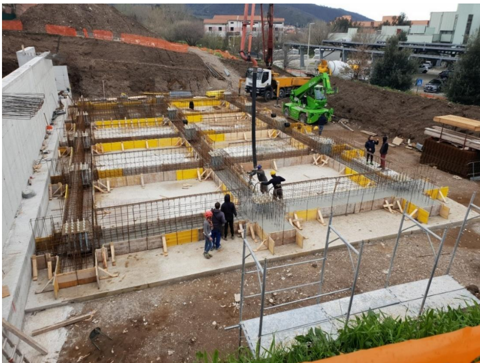
Figure 6.14 – Concrete casting of the larger base of the inverted foundation beams
