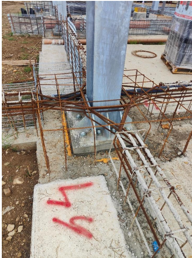
Figure 6.23 – Additional reinforcement for the completion of the foundation
