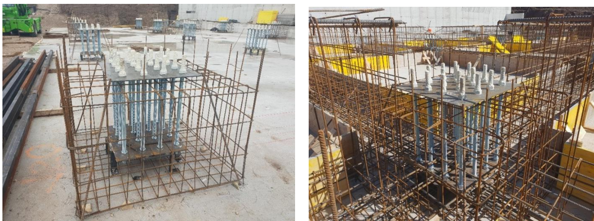
Figure 6.12 – Foundation reinforcement
