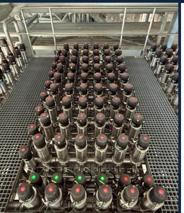
Stainless pipework for food & beverage lines, utilities and cooling (glycol/ethanol) delivered welded or press-fit.
