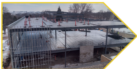
2022 - 2024 - Original costs increase due to inflation and unforeseen constructions costs for the foundation.
