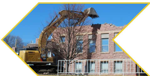
2022 - 1910 Building demolished after determination to build new building.
