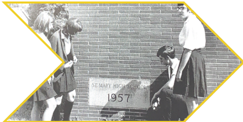
1957 - St. Mary's High School was built.
