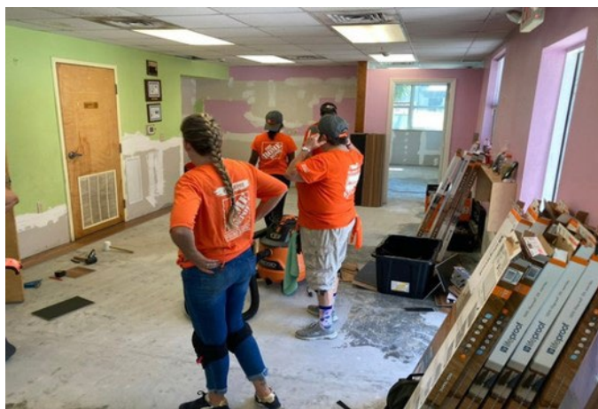
Home Depot Volunteers restoring interior
