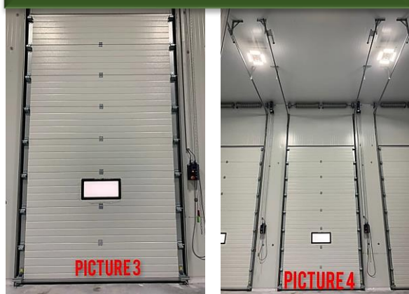
PICTURE 3 & 4 : VIEW FROM INSIDE
