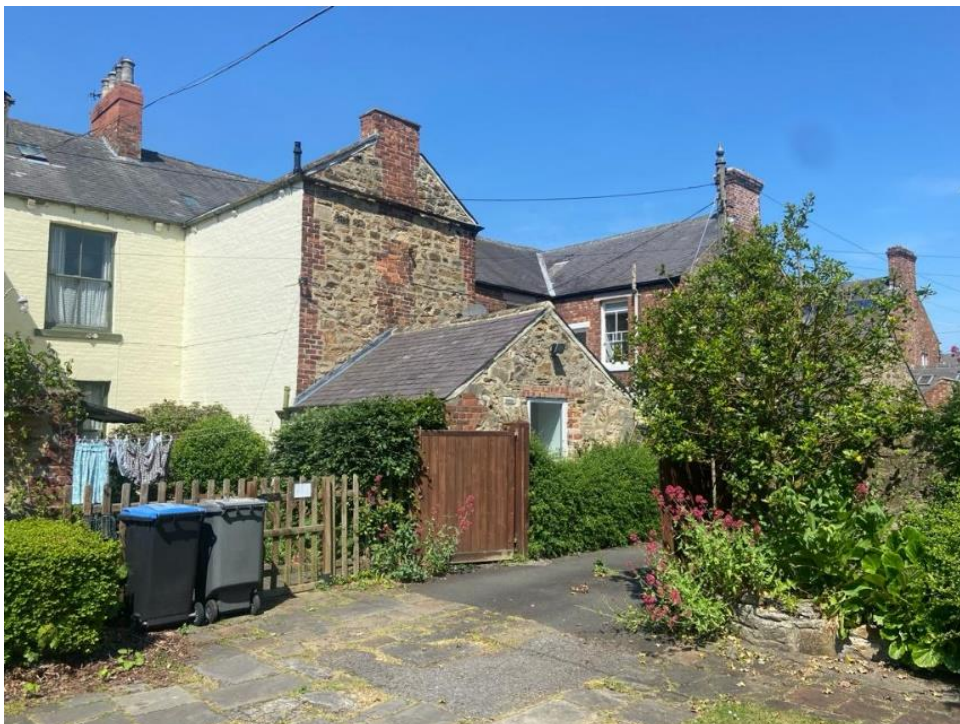
Fig 7: the stonework from the miners' cottages used in the construction of Wood View.
