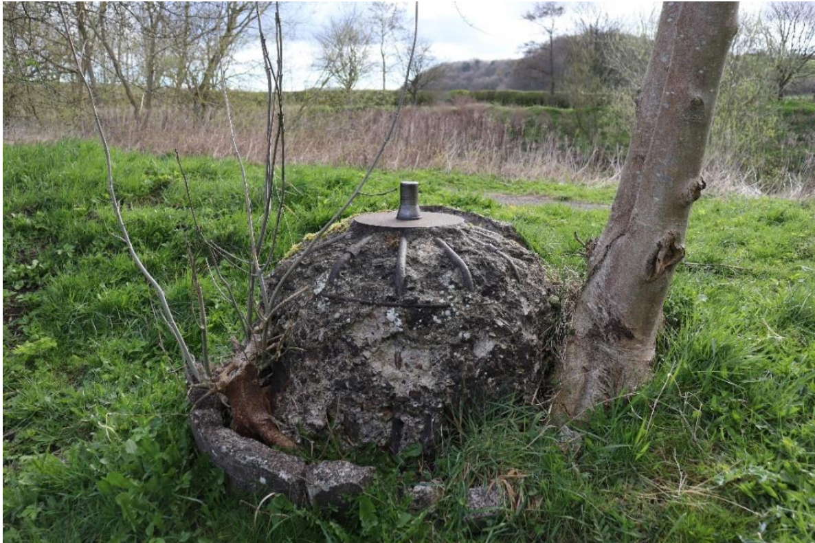
Fig. 4: The Spigot Mortar base near Shincliffe Bridge - showing the steel baseplate and pivot. Also visible are re-enforcing rods partly embedded in the now crumbling concrete.
