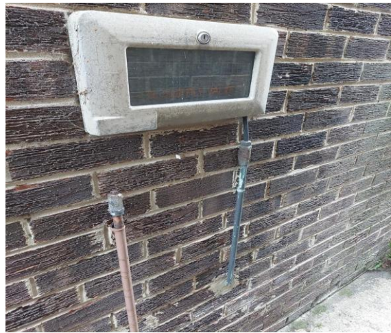
An old oil meter on the side of a house
