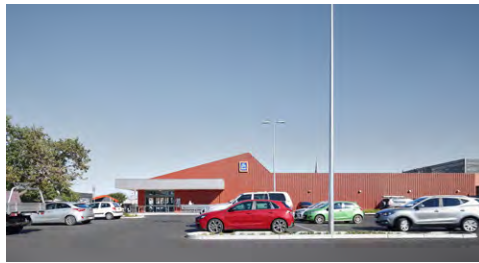
Echuca Aldi Carpark Upgrade
