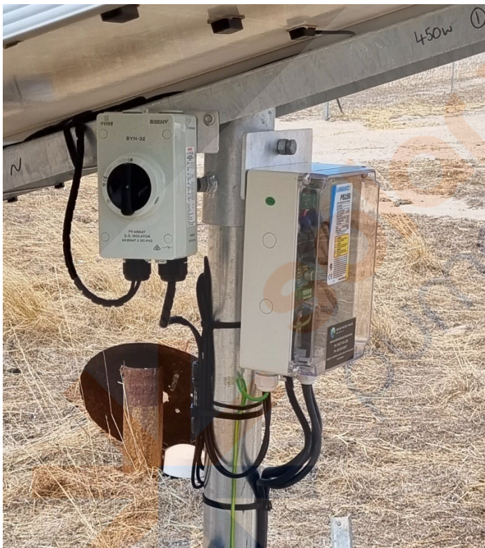
Figure 2.0 Controller installation for single panel. 1. Waterboy 2. Lorentz with Isolator.
