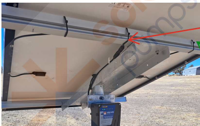
MC4 Connection to Controller
