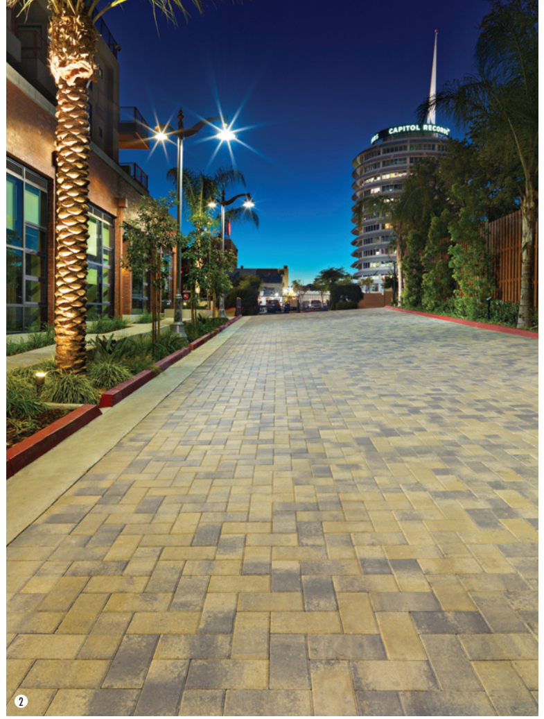
1. Holland in Gray-Charcoal installed in a 45 degree herringbone pattern. Note: This stone was manufactured at 80mm due to site conditions and anticipated traffic loads. 2. Gray-Moss-Charcoal Holland installed in a herringbone pattern. Note: This stone was manufactured at 80mm due to site conditions and anticipated traffic loads. 3. Cream-Brown-Charcoal Holland installed in a running bond pattern with a solid Mocha Holland border at the landscape edge.
