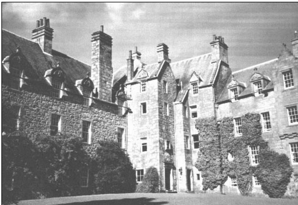
Below: Exterior view of Blair House showing entrance door (left). (Courtesy of Edward P. Blair, Blair Society of Genealogical research, Brownsburg, Indiana, USA, 1997.)
