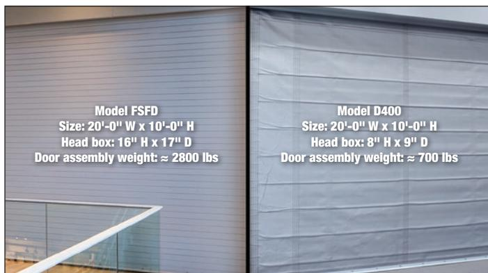
*\*Note: This curtain shutter is an opening protective in accordance with the requirements of Section 716.2 of the IBC and is NOT restricted to the language in Section 716.4 of the 2021 IBC wherein Fire Protective Curtains are tested without hose stream in accordance with UL10D and are limited to 20 minutes or less.*
