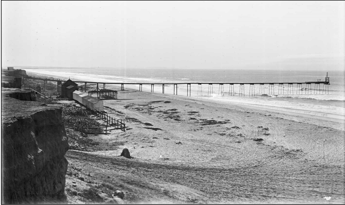
Figure 7: Construction of second pier at Oceanside (1894 - Note wide sandy beach).
