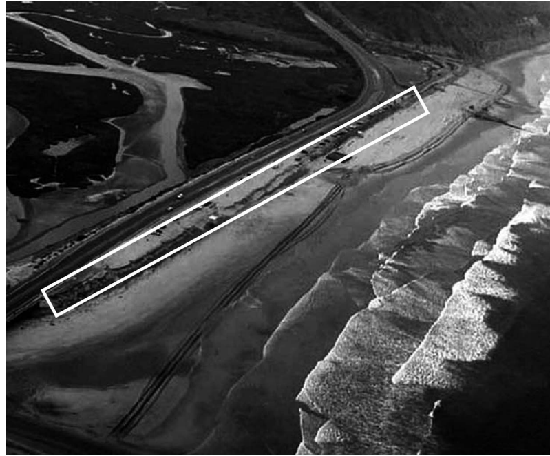
Figure 5. Approximate extent of fill on the back beach at Torrey Pines State Beach in 2001 during RBSP I (Seymour et al. , 2005).
