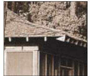
Exposed plumb cut rafters
