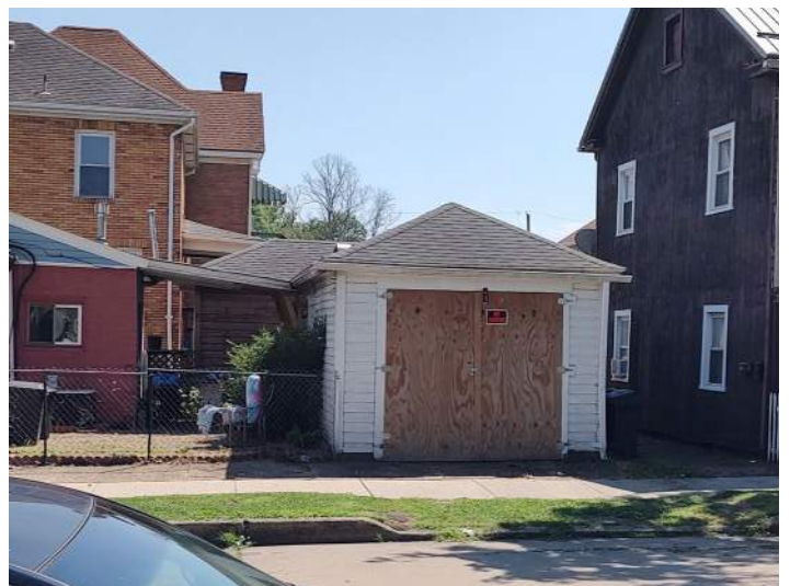
Accessory structures include garages and sheds.
