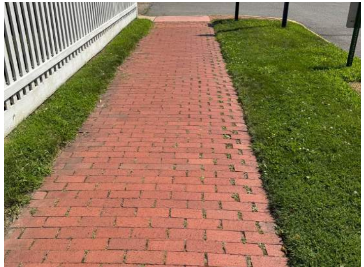
Existing paver sidewalk
