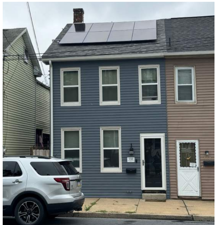
Example of inappropriate solar panel installation on roof slope easily seen from a right-of-way along the primary elevation.
