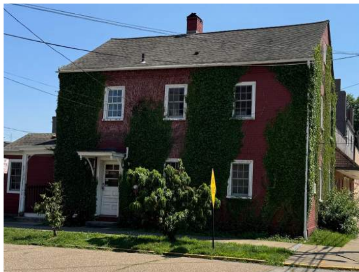
Detached residential building in the Economy Historic District.
