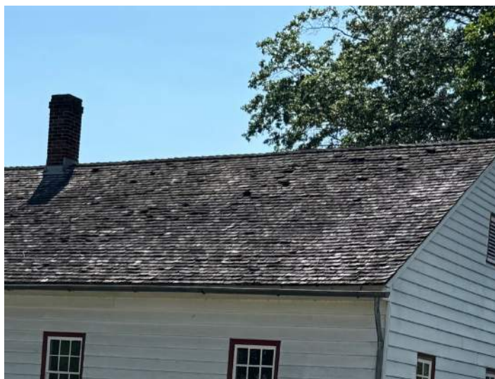
An example of wood shingle roofing.
