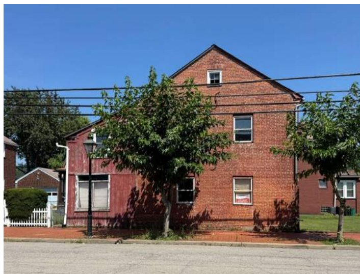
Detached residential building in the Economy Historic District.
