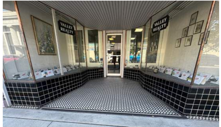
Recessed storefront with wood panels, detailing, and signboard.
