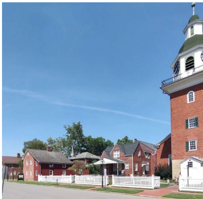
A building's setting includes its relationship to other elements, such as any front yards, sidewalks, streets, and geography.
