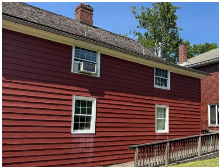
An example of wood siding on a Harmonist structure
