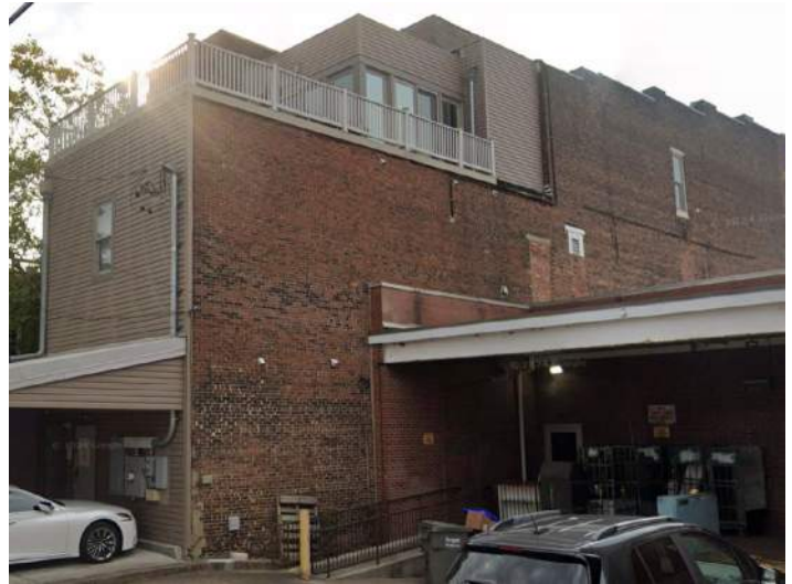
Addition and roof deck appropriately located at the rear.
