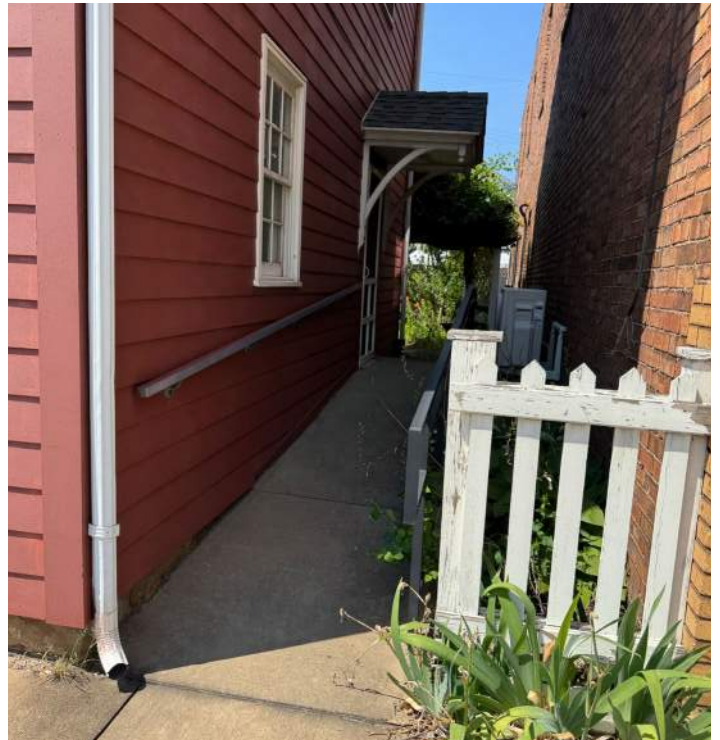
Example of an appropriate accessible entry modification.
