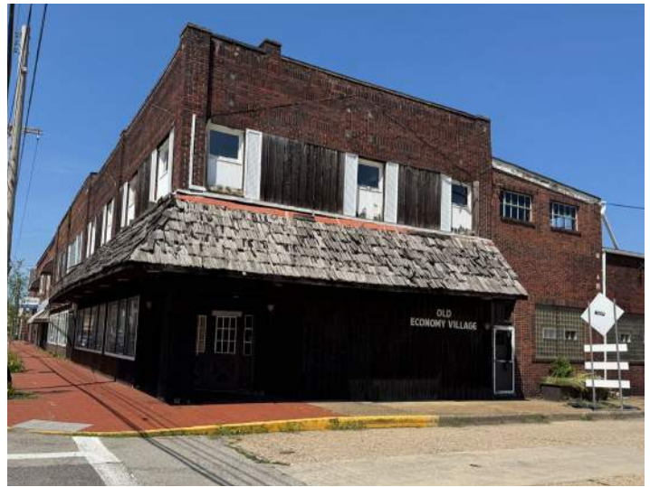
Two-story commercial building in the Economy Historic District.
