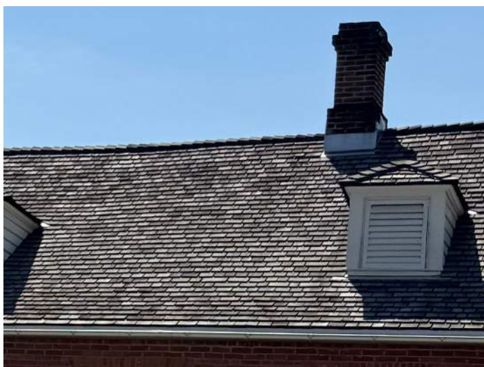
Harmonist structures were originally built with wood shingles.
