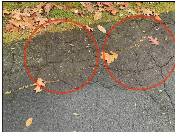
41. Cracked or damaged surfaces. Recommend...
