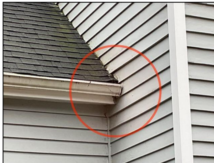
4. Kickout flashing - missing
