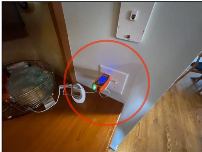
49. Recommend GFCI protected outlets for all...
