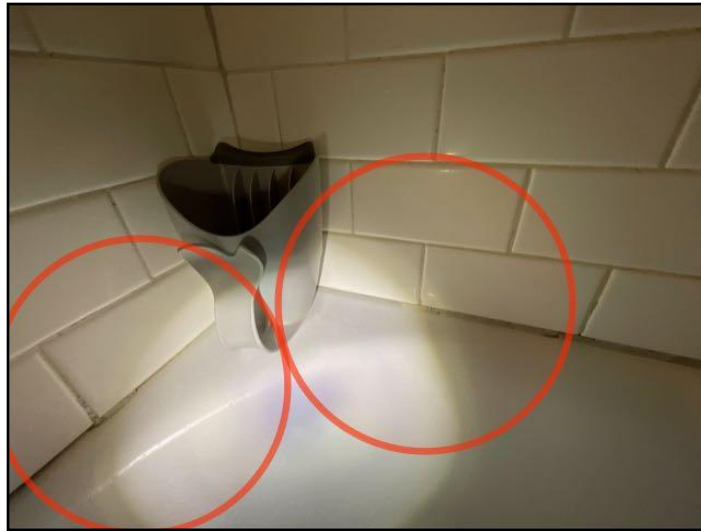
82. The caulk between the bathtub/shower and th...
