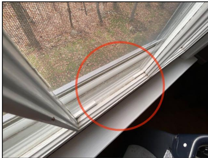
22. Putty missing, cracked or deteriorated
