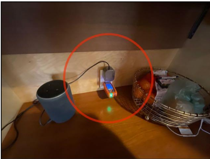
48. Recommend GFCI protected outlets for all...
