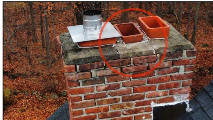
61. Cracked - The crown at the top of the...
