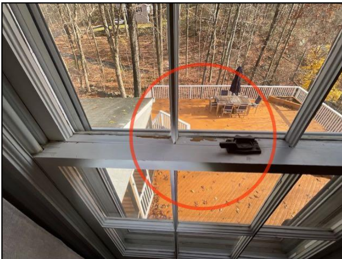
18. Putty missing, cracked or deteriorated
