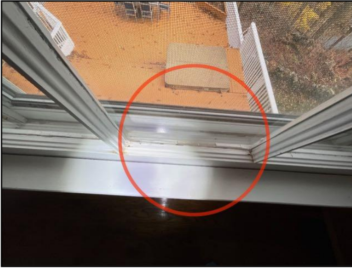
20. Putty missing, cracked or deteriorated
