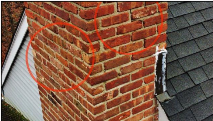
62. Spalling/Loose Bricks
