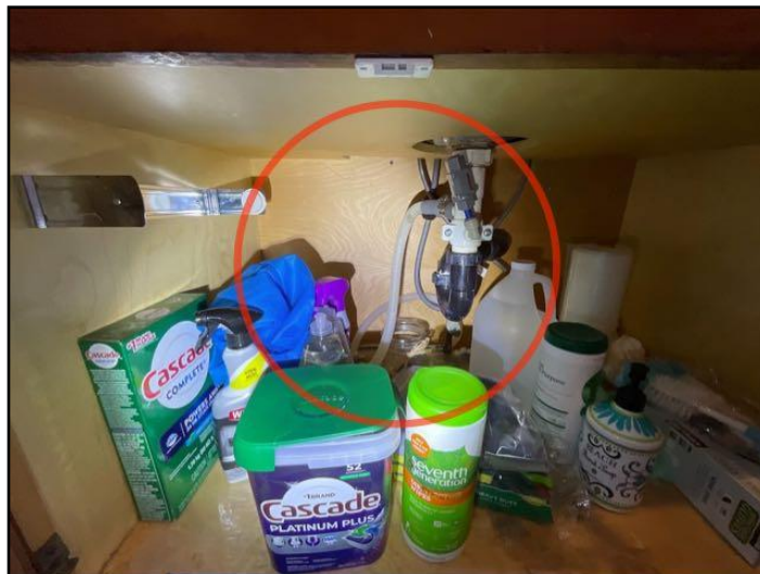
94. Backflow prevention high loop missing
