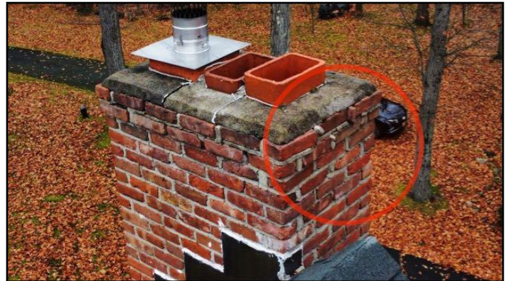
63. Spalling/Loose Bricks
