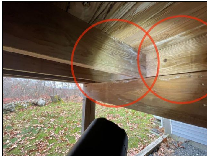
34. End bearing inadequate
