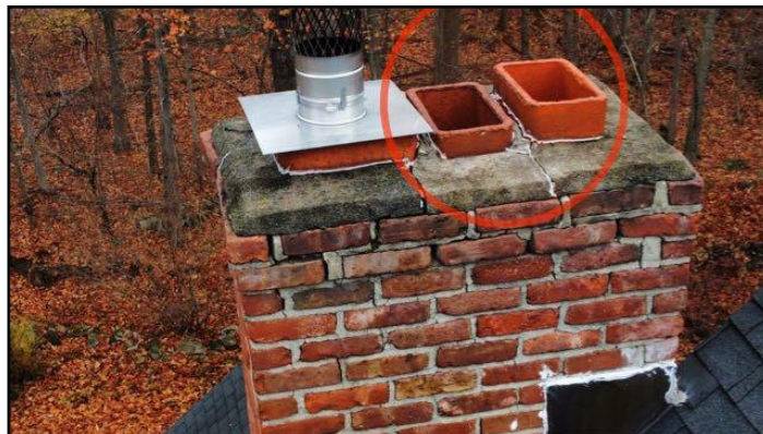
64. Rain cap missing or damaged
