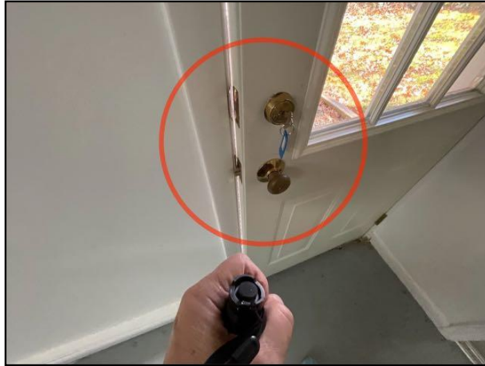
88. Door lock was controlled by a key turn...
