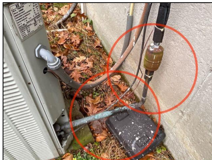
67. Insulation - missing
