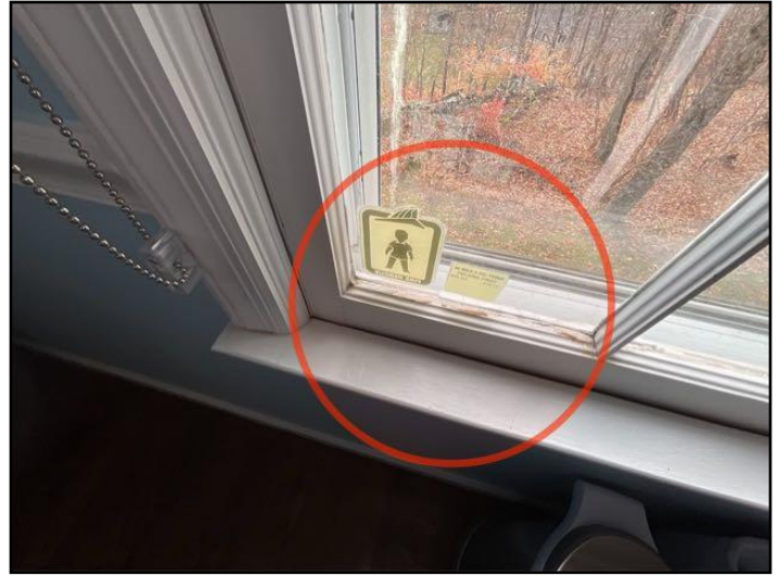
21. Putty missing, cracked or deteriorated
