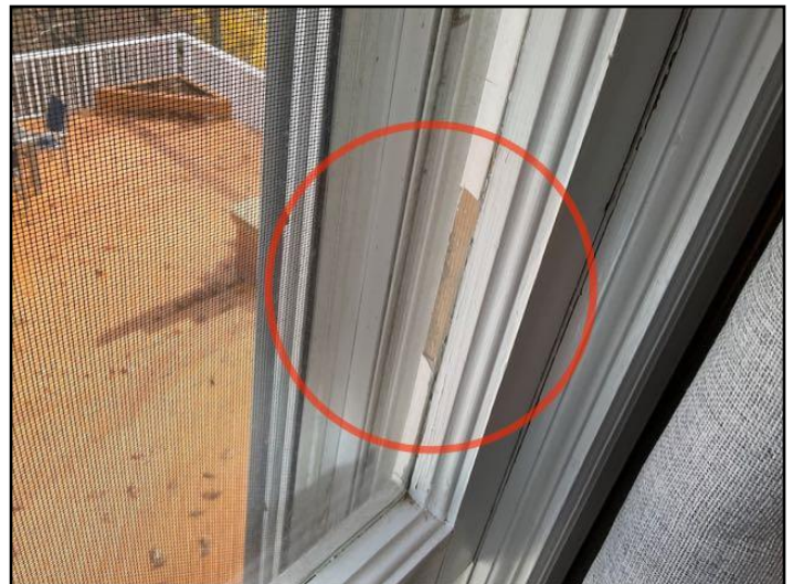
19. Putty missing, cracked or deteriorated
