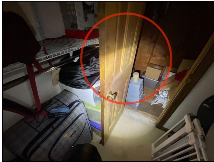
74. The knee wall door was not insulated....
