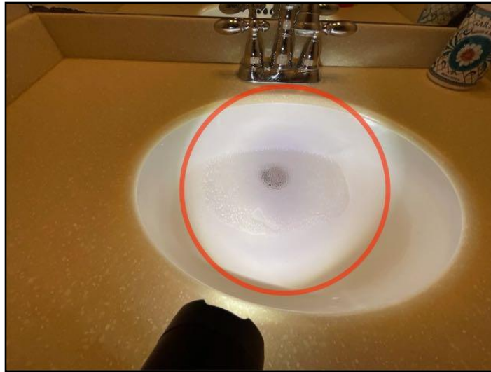
78. Slow drain. Recommend snaking the drain or...
