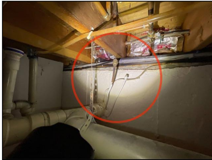
65. Copper oil lines were observed coming...
