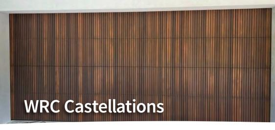
This is a vertical 81x26mm Western Red Cedar Screen Clad. This style is available in Screen Clad or Castellations profile in either 18mm or 26mm thick. The timber is fixed to a black powder coated frame.
