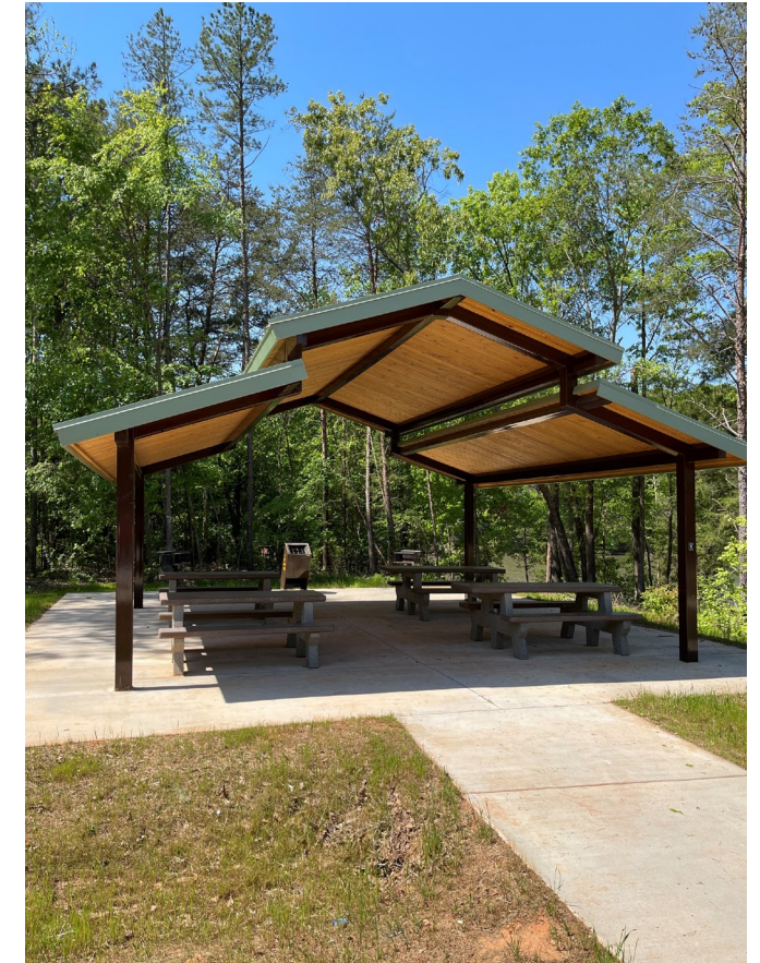
Springs Park Picnic Shelter
