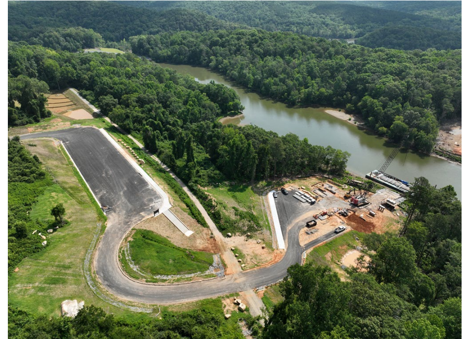
Lower Great Falls Canoe/Kayak Access and Pedestrian Bridge Site Construction
