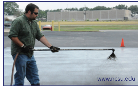
Applying sealant to a parking lot.
