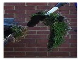
Your carbon poles are extremely strong. However avoid over straining/bending them when handling heavy grass deposits when cleaning 6 plus poles high. Best practice to remove heavy tufts of grass from gutters is chop down to manageable lengths.
