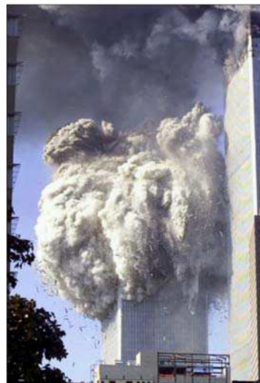
The collapse of WTC building Two.
